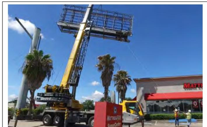
*The proposed Project would involve the demolition of the existing pole sign structure and would include the use of a hydraulic truck crane and other heavy equipment during the construction and installation of the proposed digital sign.*
