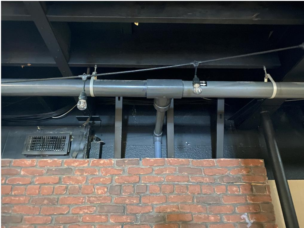
Photograph 20. Example of SSDS piping (06/01/2021).
