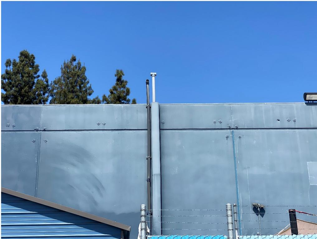
Photograph 45. Effluent air stack, part of the SSDS (06/01/2021).
