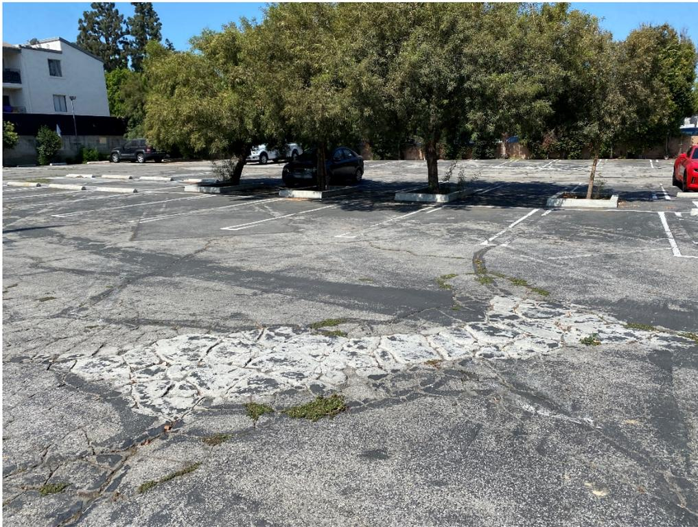
Photograph 33. Asphalt pavement in the southern portion of the Site, in poor condition (06/01/2021).
