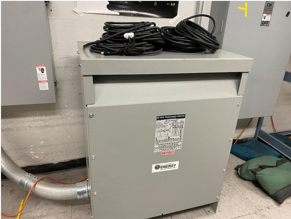
Photograph 14. Small dry-type electrical transformer located in the equipment room (06/01/2021).
