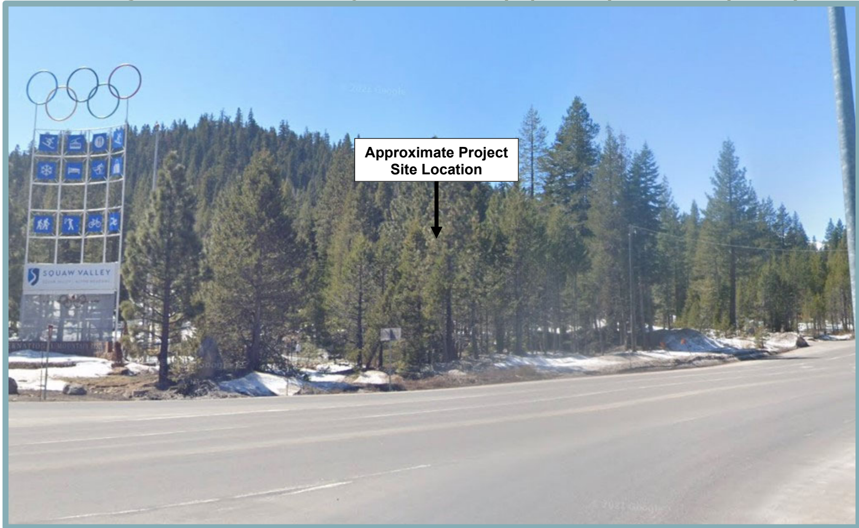
Figure 4-4 Existing Views Towards The Project Site From Olympic Valley Road West (View 2)
