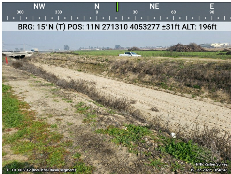
Figure 4. P-10-005812 at location of Industrial Basin pipeline tie-in.
