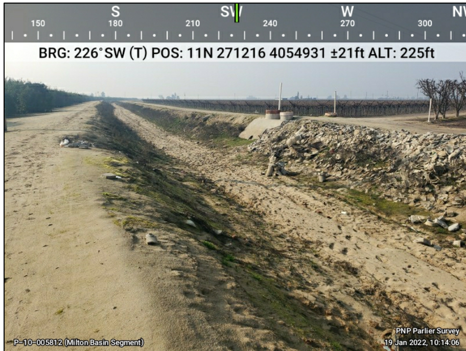
Figure 3. P-10-005812 at location of Milton Basin pipeline tie-in.
