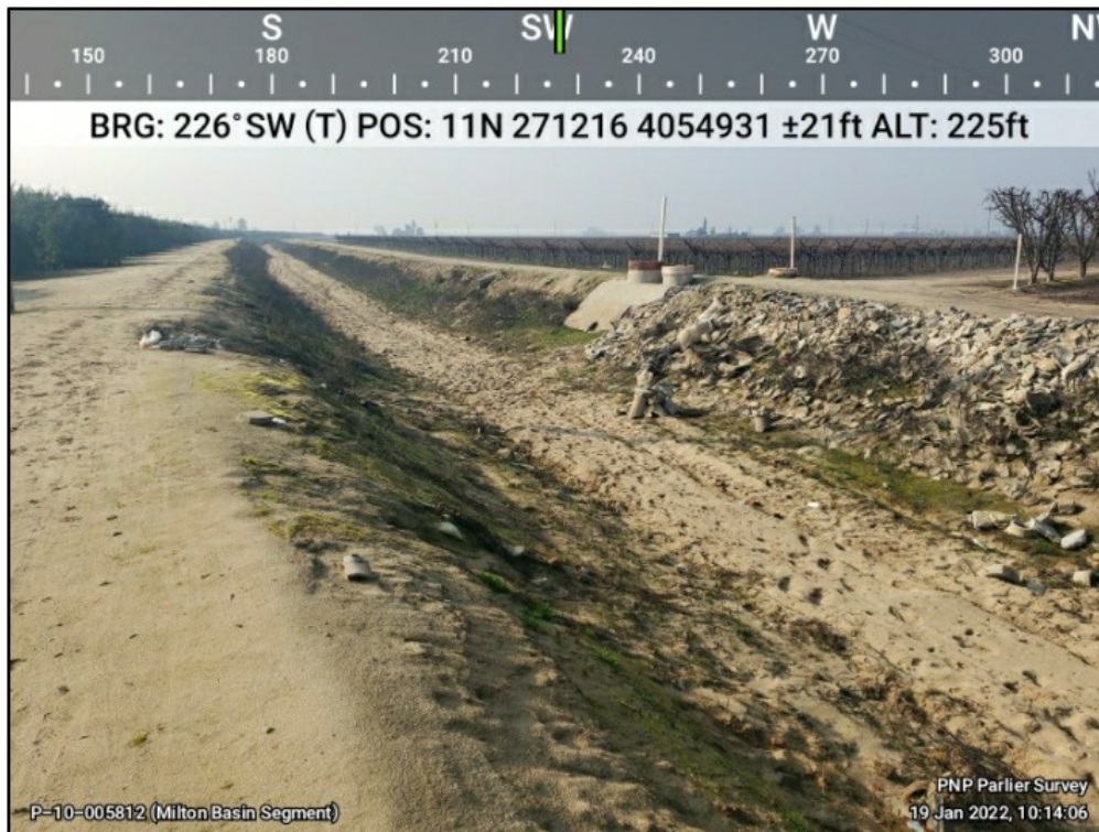
Figure 4-5: Centerville-Kingsburg Canal (P-10-005812) at location of Milton Basin pipeline tie-in.
