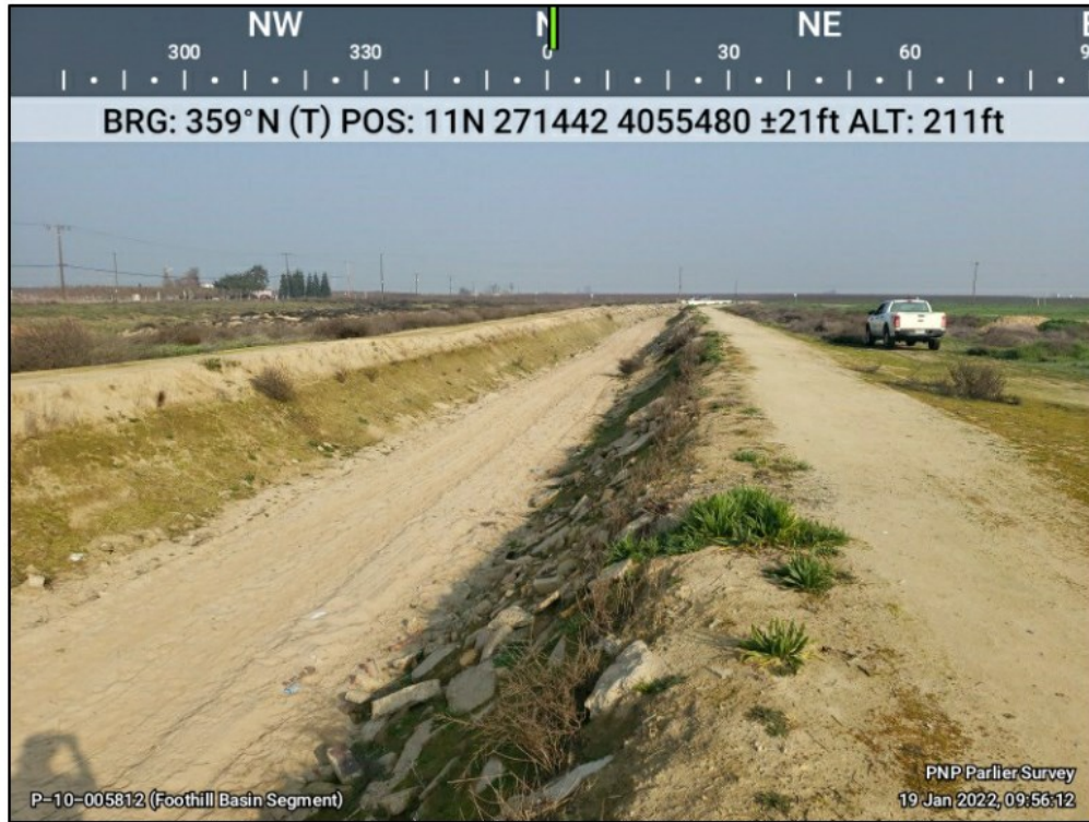
Figure 4-4: Centerville-Kingsburg Canal (P-10-005812) at location of Foothill Basin pipeline tie-in.
