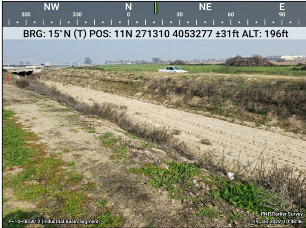
Figure 4-6: Centerville-Kingsburg Canal (P-10-005812) at location of Industrial Basin pipeline tie-in.
