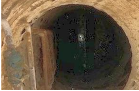
Manhole Before Install
