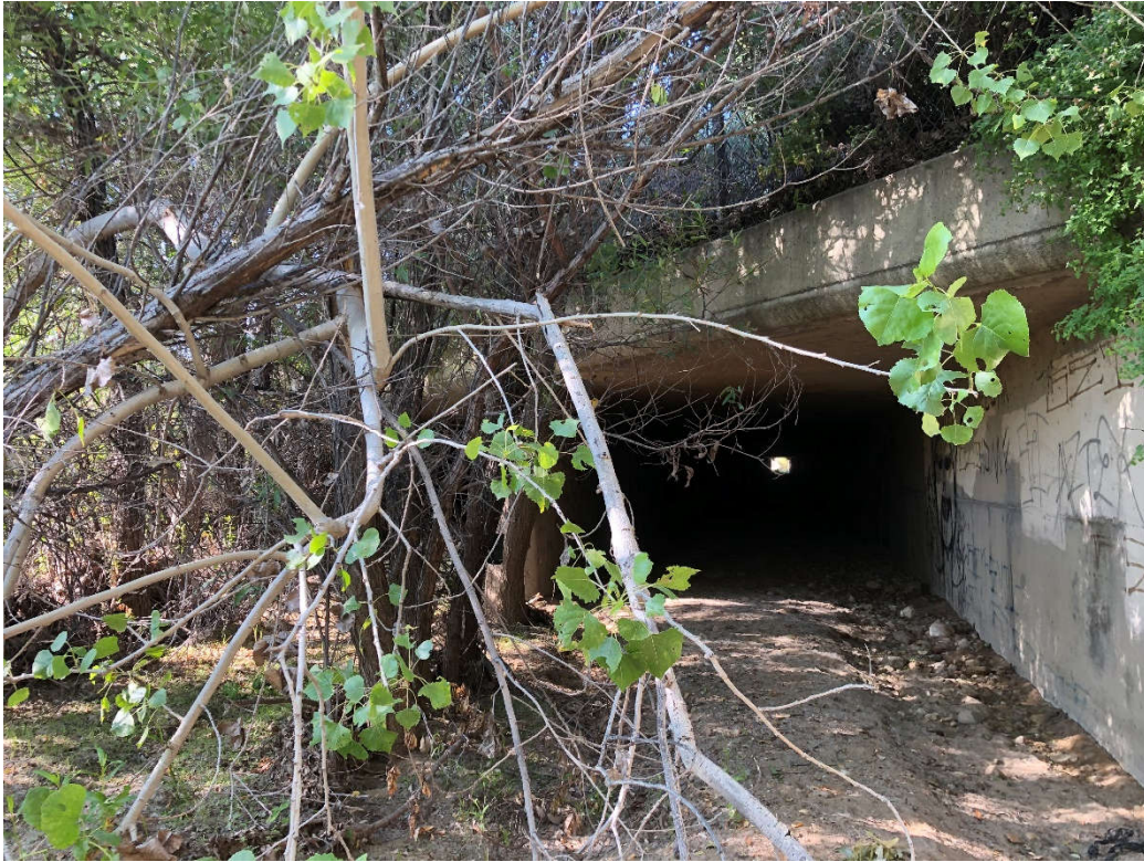
Photo 1 –Culvert crossing of IS-1 under I-5, facing southwest (6/3/20).
