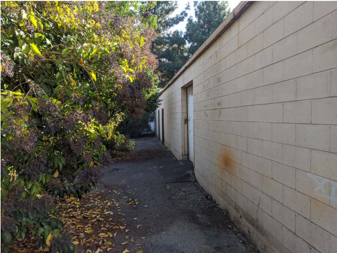
Photograph 4 - View of the northeastern side of the Property
