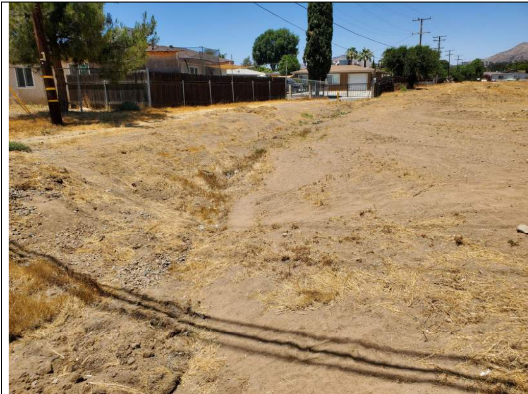
Photo 13. Ephemeral swale that receives stormwater runoff from Watson Way to the roadside swale that parallels the north side of Cottonwood Avenue; looking north from southwest corner of Subject Parcel.
