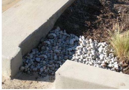
Figure 2: Curb Cut located in a Bioretention Facility
