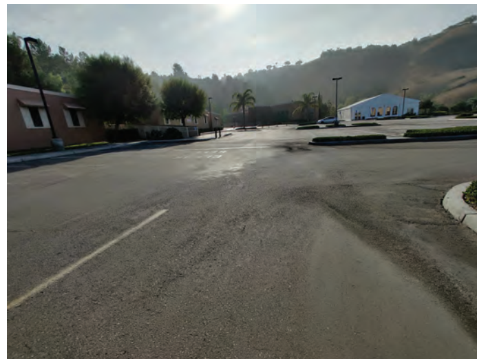
PARKING LOT #1 LOOKING WEST
