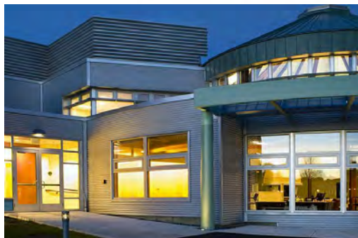
B REAR ADDITION EXTERIOR CLADDING & ENTRY CANOPY, TYP: MBCI "PBC" HORIZONTAL CORRUGATED METAL PANEL IN "GALVALUME" CORRUGATED METAL PANEL
