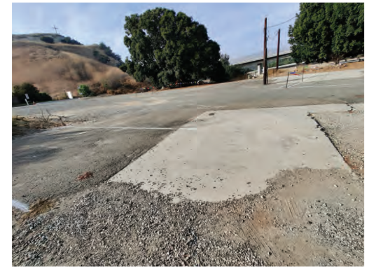
PARKING LOT #6 LOOKING NORTH
