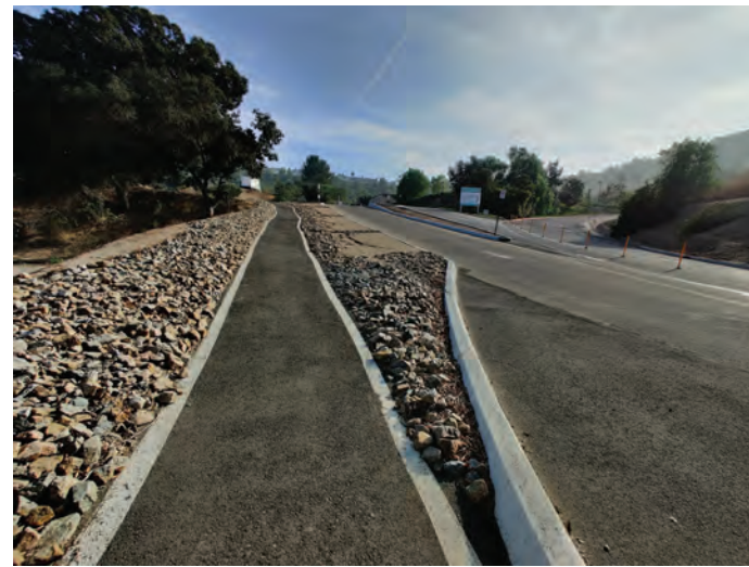
PEDSTRIAN PATH FROM SITE ENTRY LOOKING SOUTH
