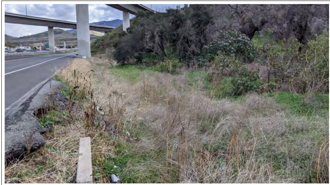
Photo of the roadside ditch located along the northern boundary of the project site south of East Santa Ana Canyon Road.
