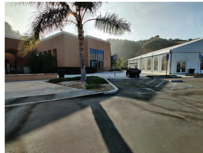
MAIN AUDITORIUM AND FABRIC BUILDING LOOKING WEST
