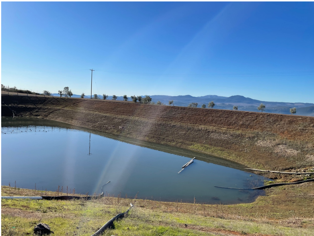
20-acrefoot Off-stream Water Storage Reservoir (south view)
