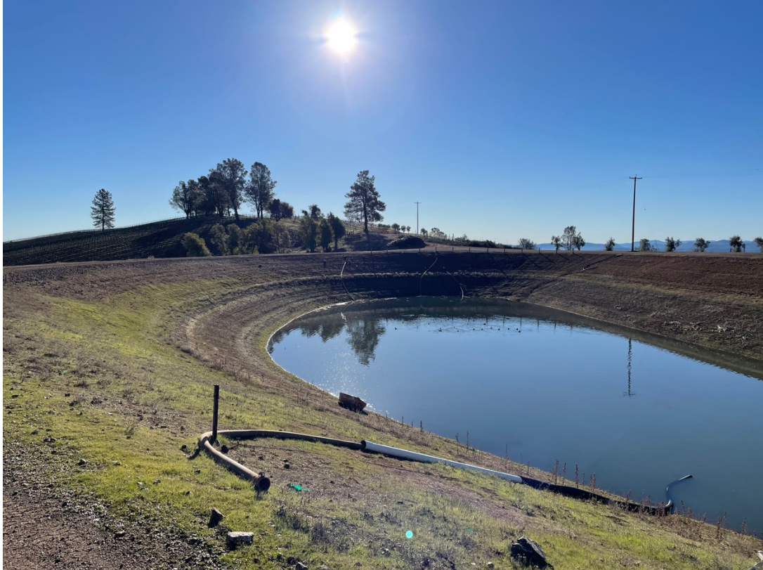
20-acrefoot Off-stream Water Storage Reservoir (southeast view)
