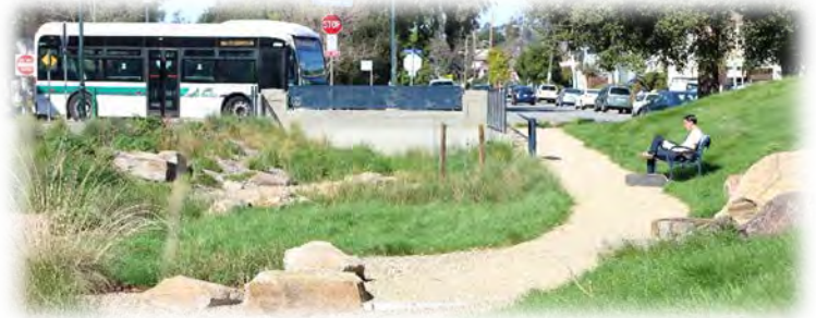
Bioretention facility in El Cerrito with active and passive recreational uses.
