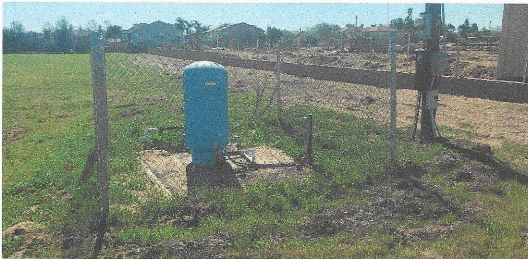
Photo 2B: Water-Well at 463 Honey Lane (viewing south)
