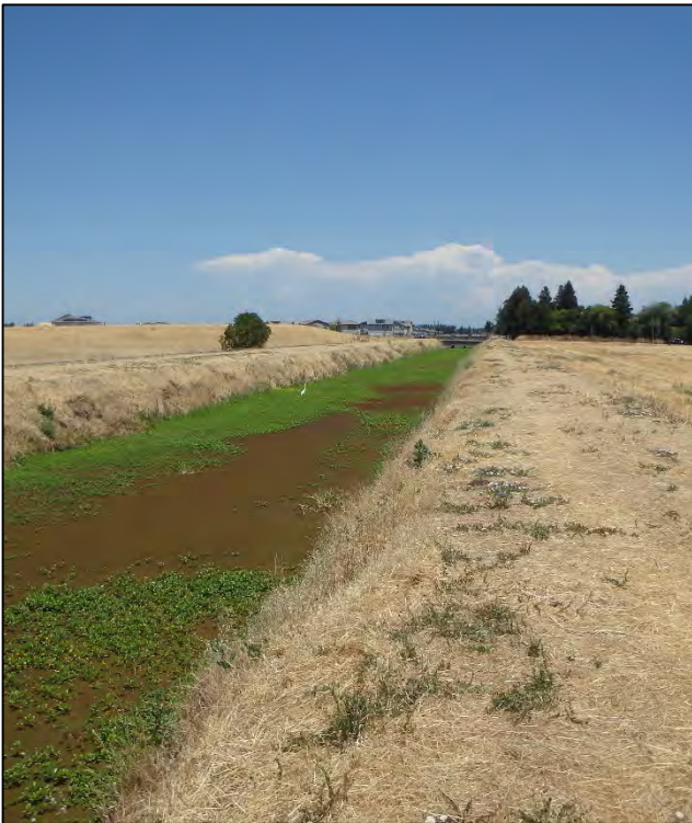
Photo 7. Drainage canal located at Well 15.
