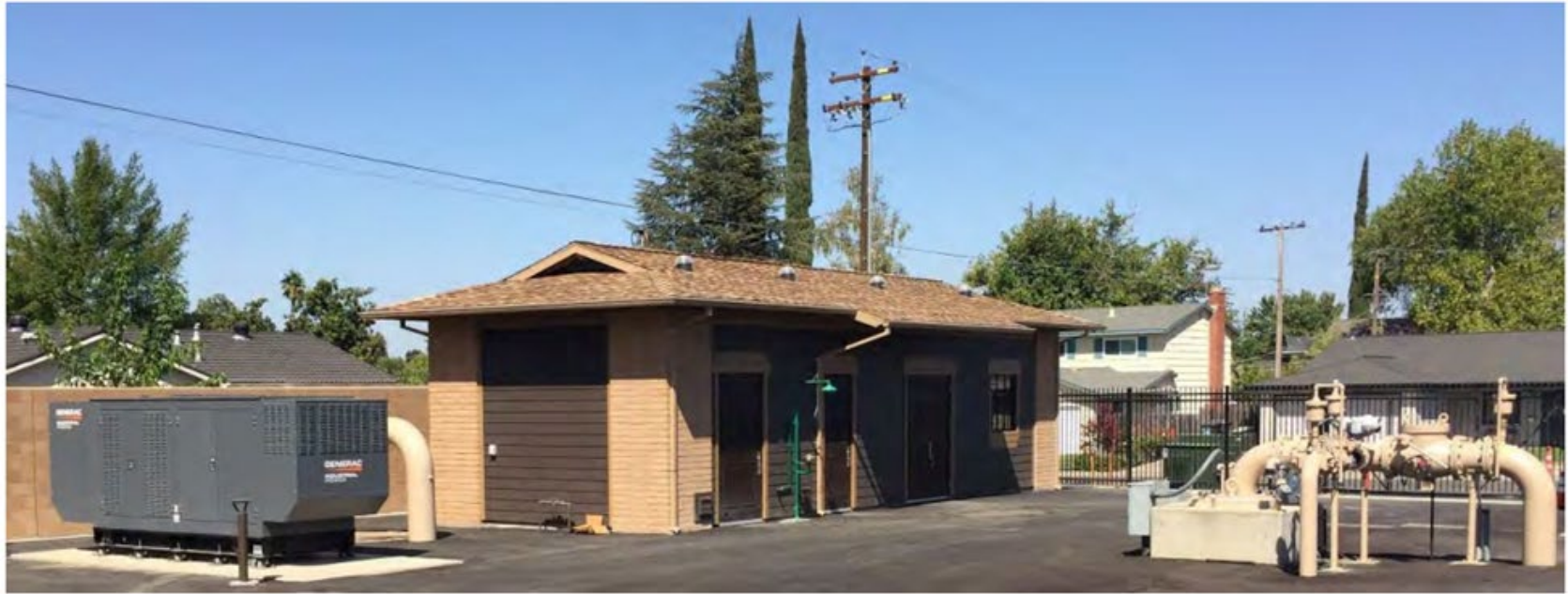
Figure 3: Example of an Existing Well Site
