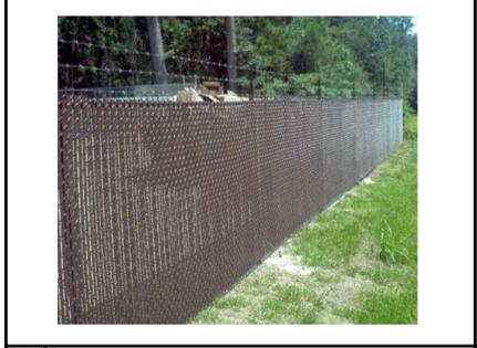
**B SLATTED CHAIN LINK FENCE WITH BARBED WIRE**
