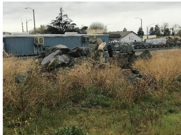
Looking Northwest – Construction Debris Pile (Mostly Rock with Some Disaggregated Asphalt, Appears to Be Staged Rip-Rap)
