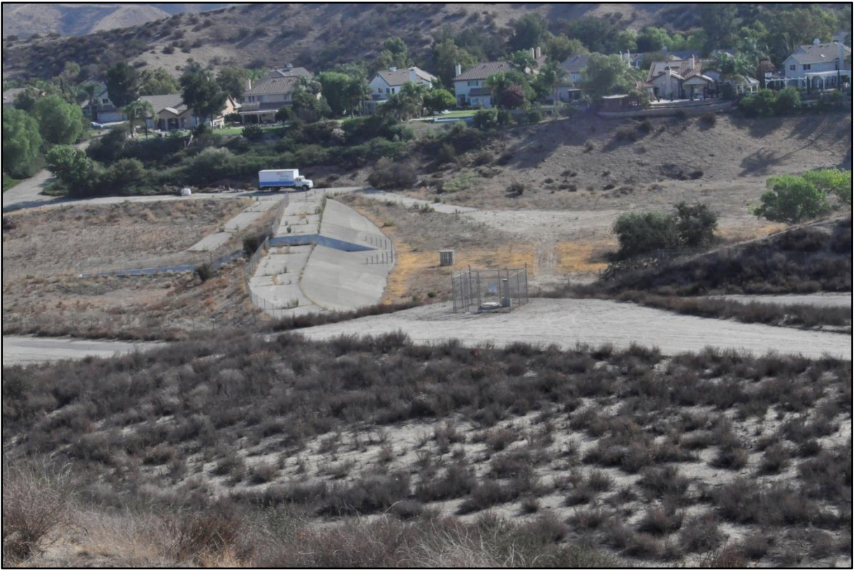
Figure 14. View towards the northwest of the water retention basin located north and outside of the current Project boundary.
