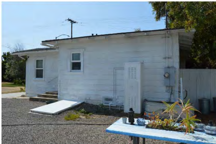
North façade, view facing southeast.
