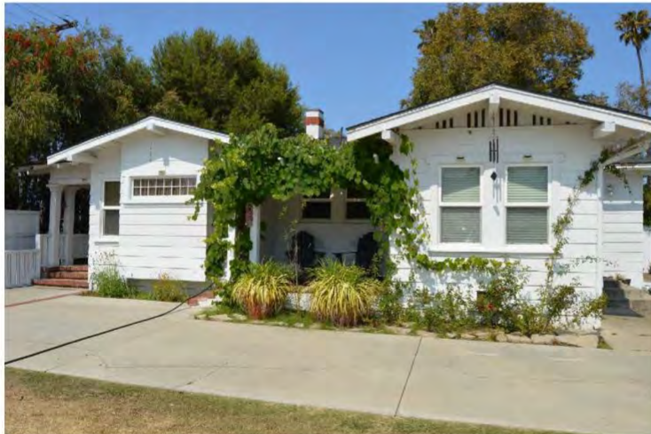
East façade, view facing southwest.
