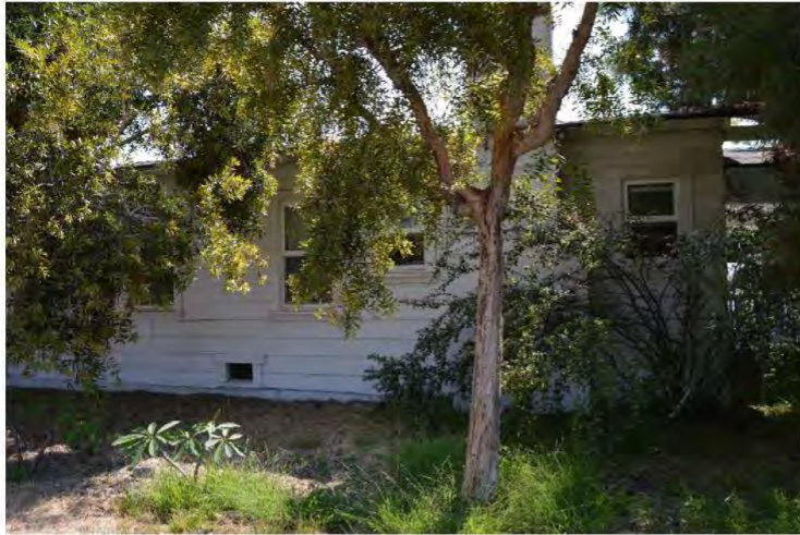
West façade, view facing northeast.
