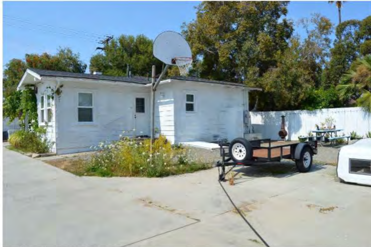
North façade, view facing southwest.
