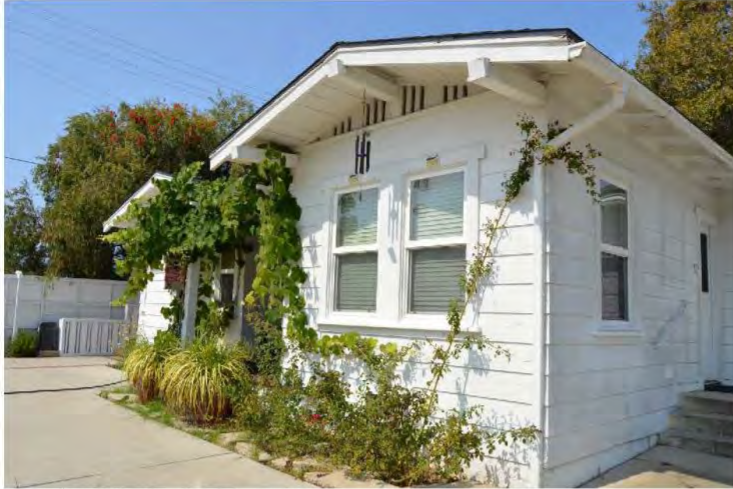
East and north façades, view facing southwest.
