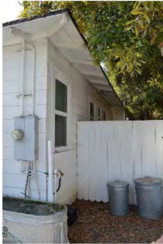
West façade, view facing southeast.
