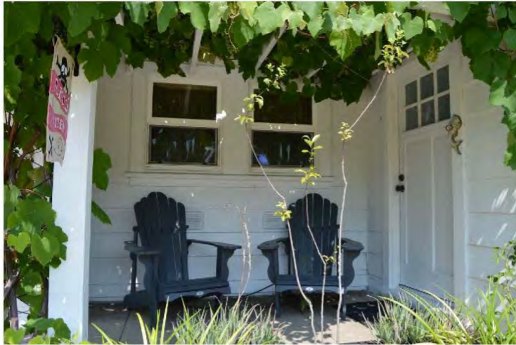
Detail view of recessed side porch and secondary entrance, facing northwest.
