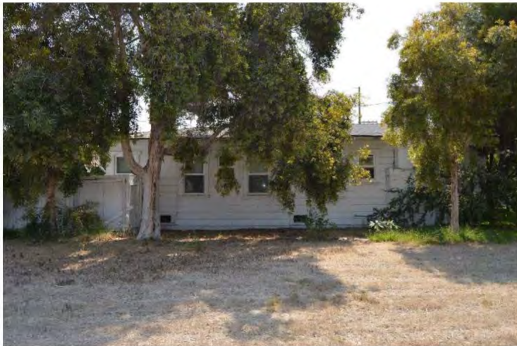
West façade, view facing east.
