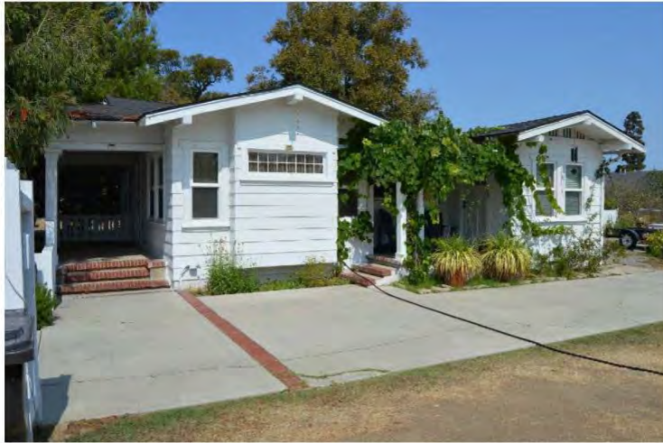
East façade, view facing northwest.
