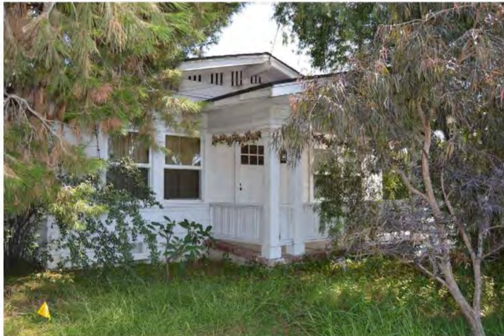
South (primary) façade, view facing northeast.
