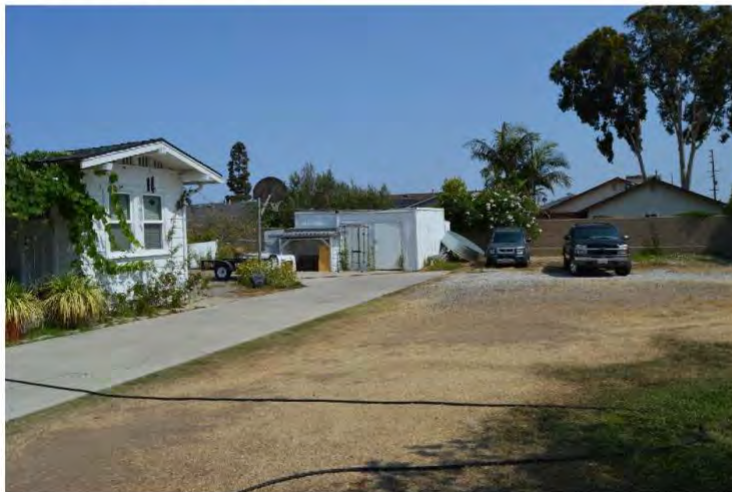
Front yard, driveway, and metal shed, view facing northwest.
