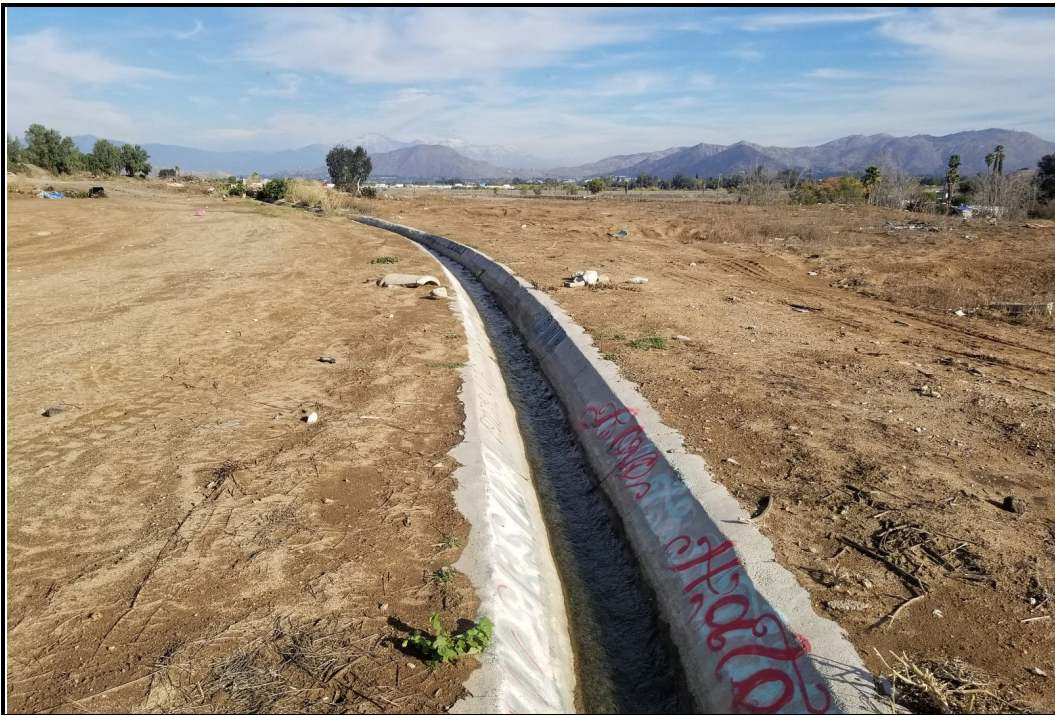
PHOTOGRAPH 2 View of Concrete V-ditch Section of Jurupa Ditch Looking South
