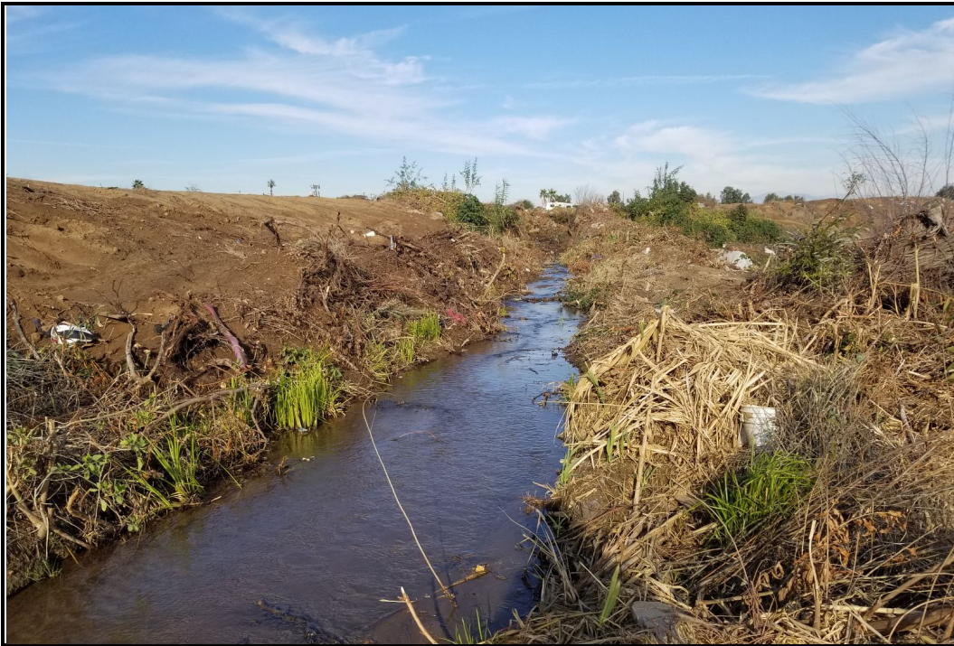
PHOTOGRAPH 5 View of Earthen Channel Section of Jurupa Ditch Looking South
