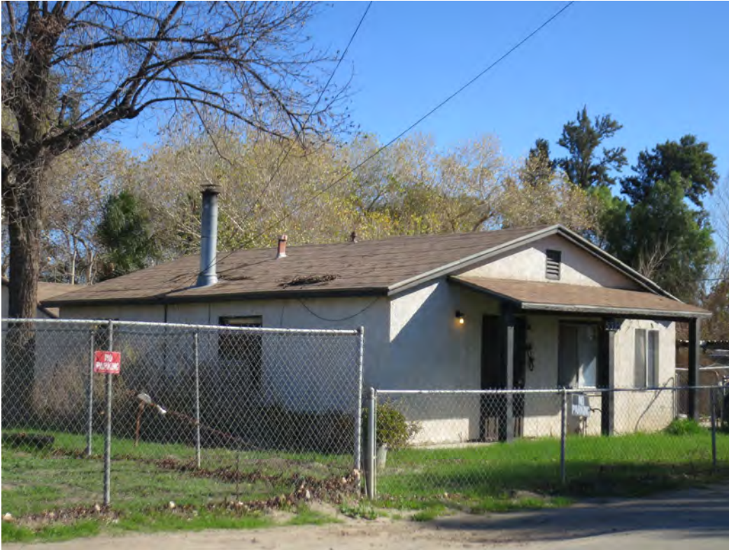
Photo 1. Oblique view of 5325 34th Street, looking northeast
