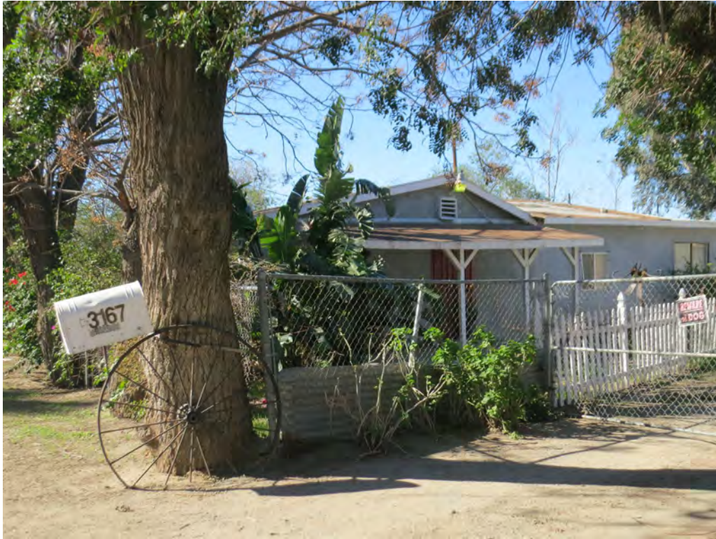
Photo 1. Oblique view of 3167 Wallace Street, looking southwest
