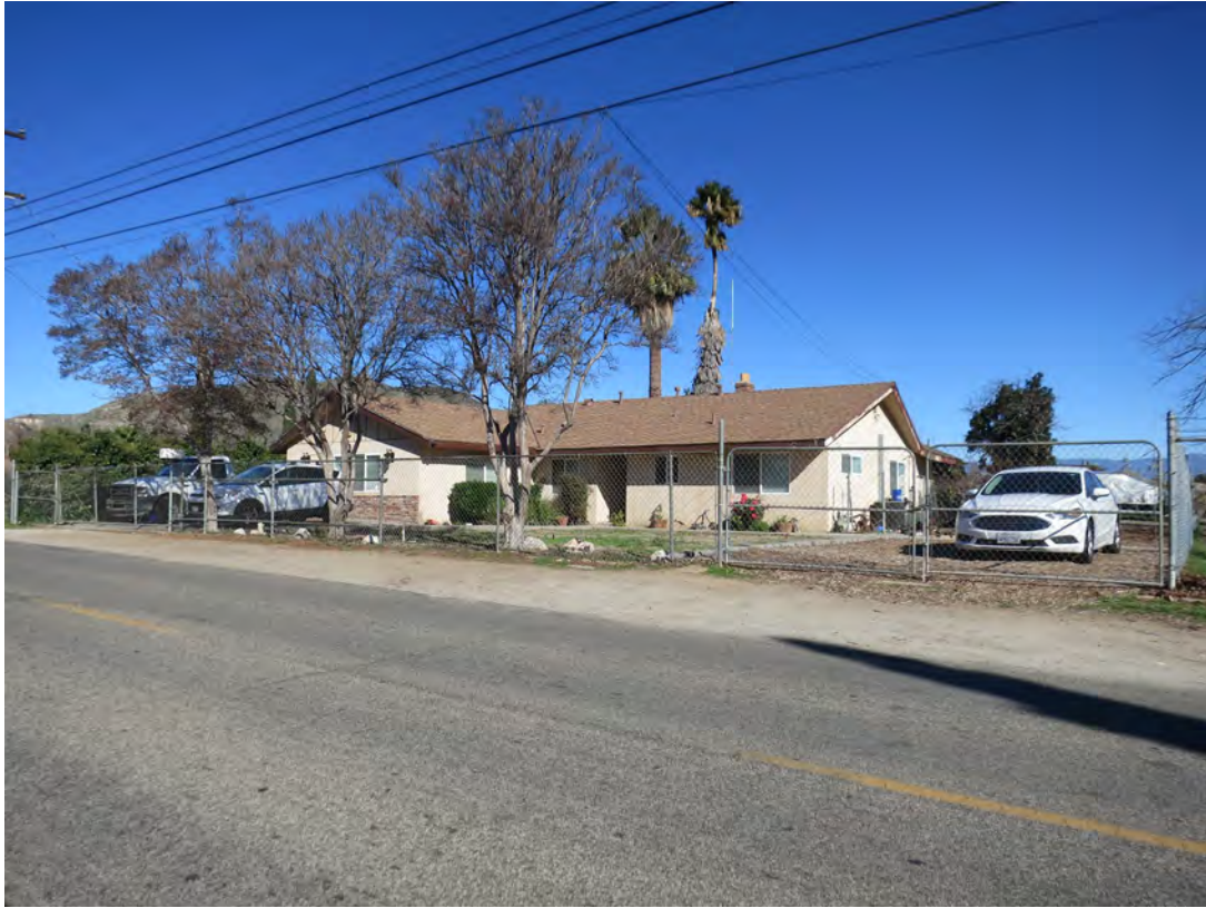
Photo 1. Oblique view of 5455 34th street, looking northwest
