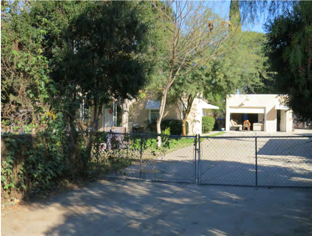
Photo 1. Oblique view of Building 1 at 5281 34th Street, looking northwest
