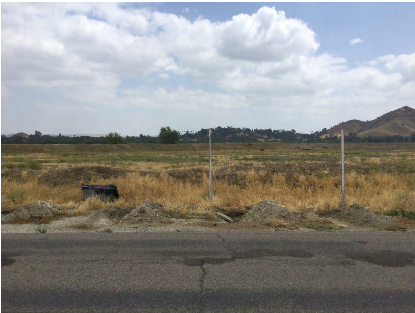
Figure 1. An overview of the previously recorded location of P-33-014347, facing southeast.
