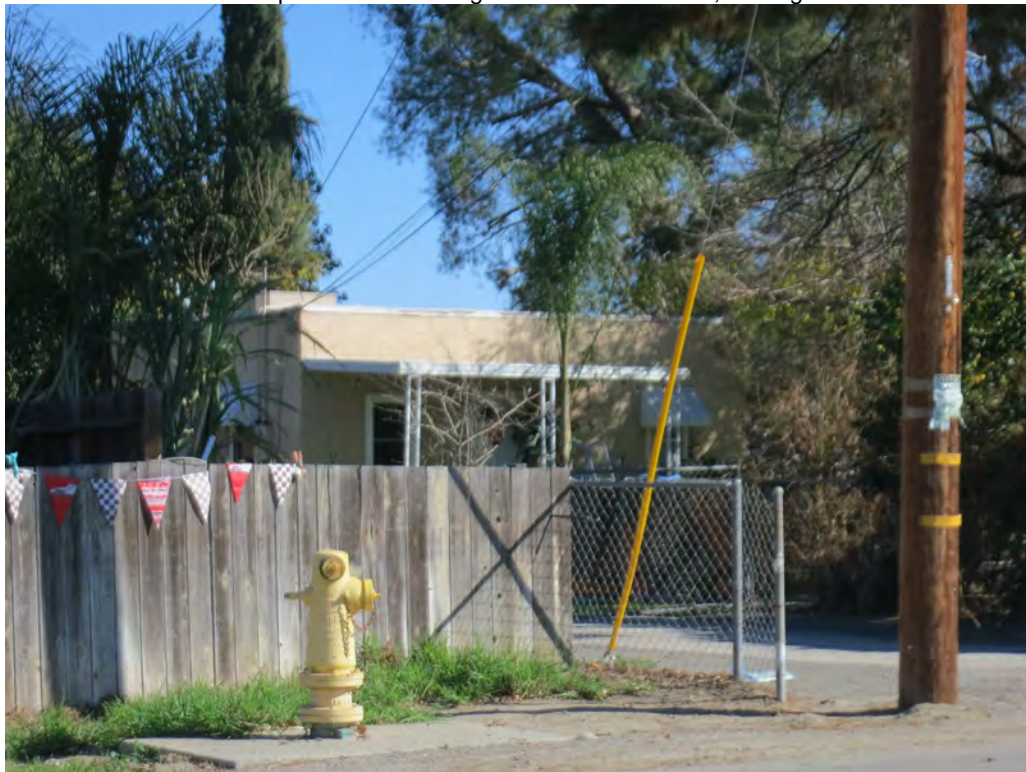
Photo 2. Oblique view of Building 2 at 5281 34th Street, looking northeast
