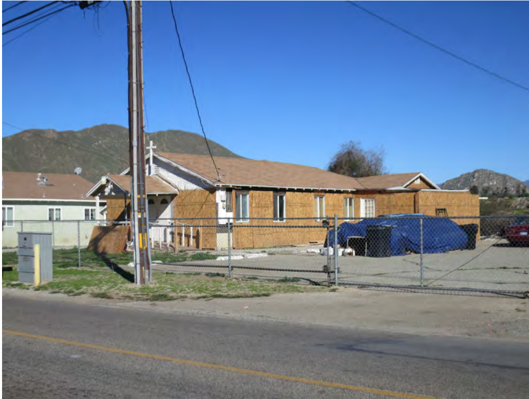
Photo 1. Oblique view of church 5413 34th street., looking northwest
