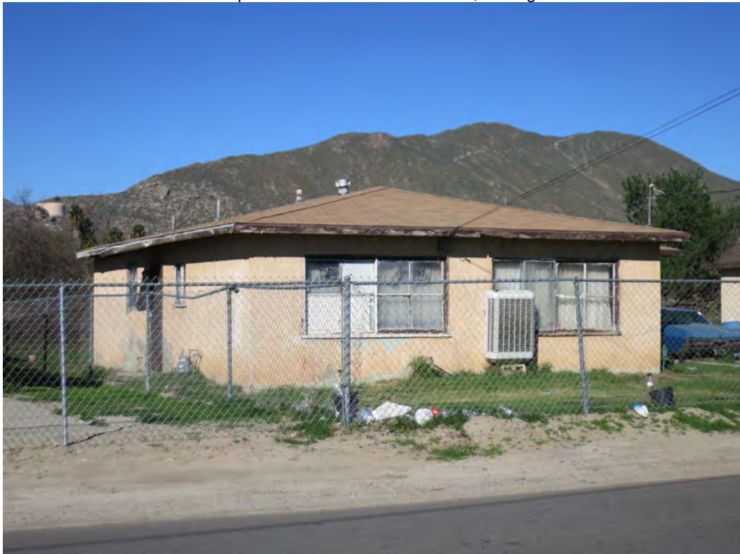
Photo 2. Oblique view of 3377 Wallace Street, looking northwest
