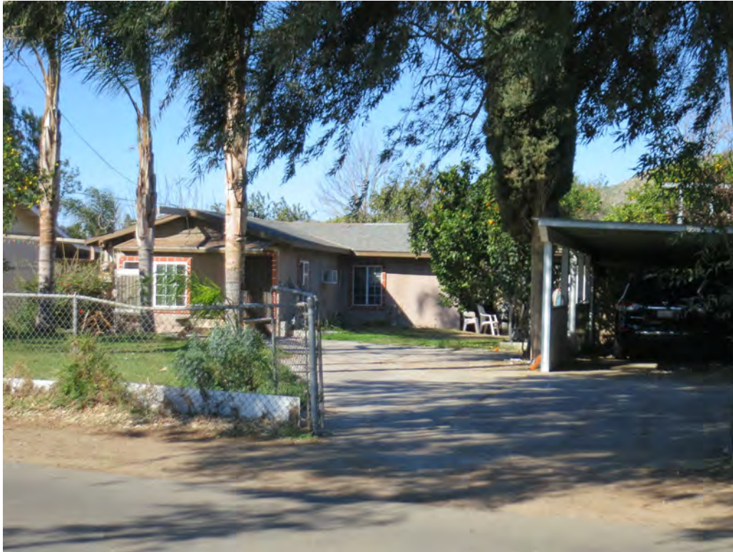
Photo 1. Oblique view of 3295 Wallace Street, looking southwest
