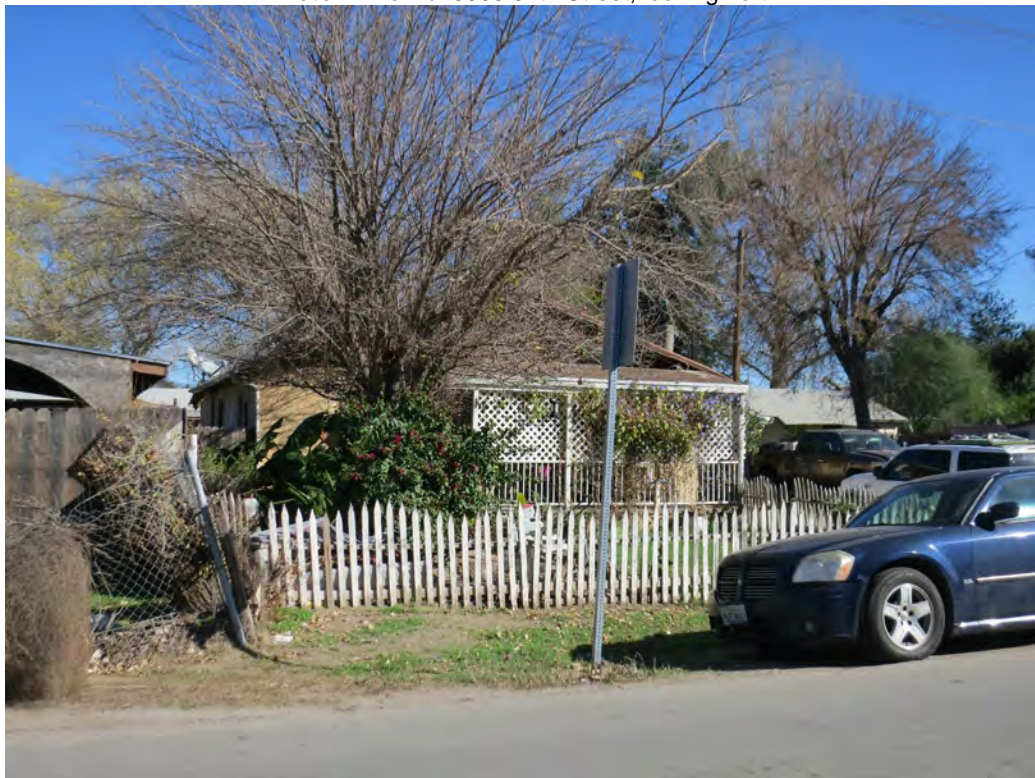
Photo 2. Oblique view of 5305 34th Street, looking northwest
