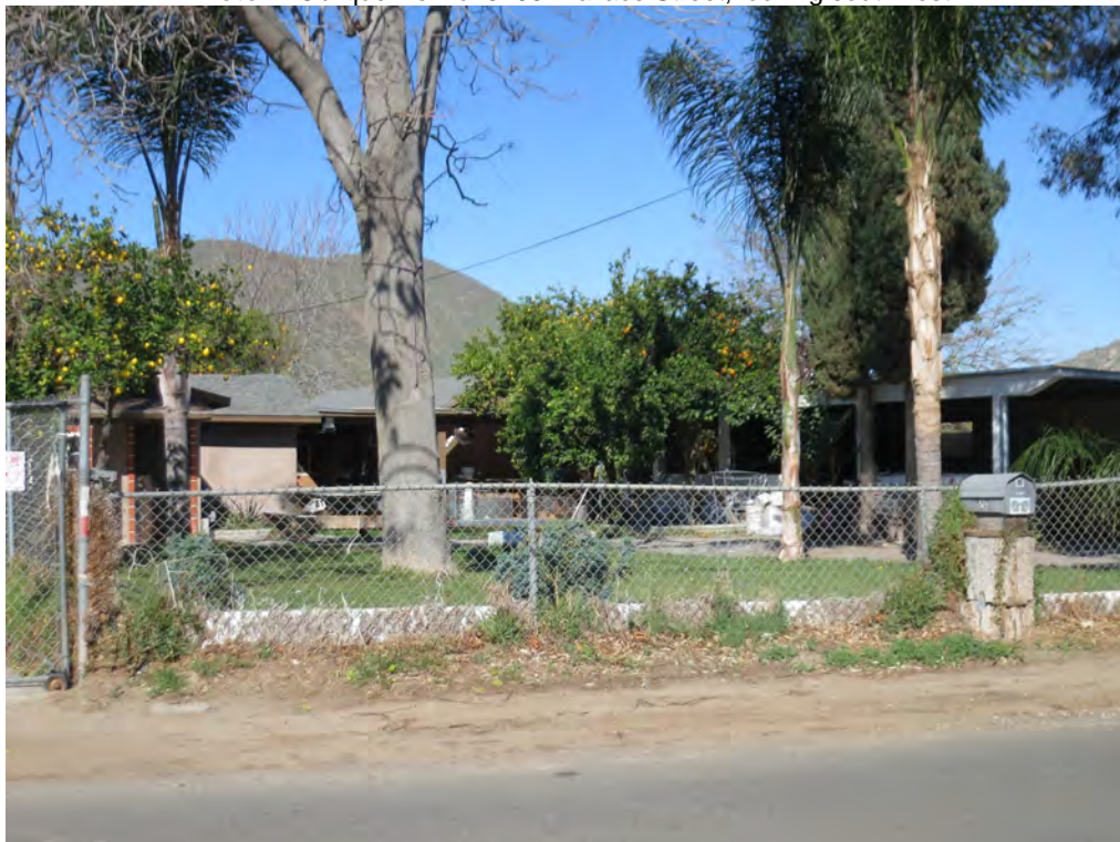
Photo 2. Oblique view of 3295 Wallace Street, looking northwest
