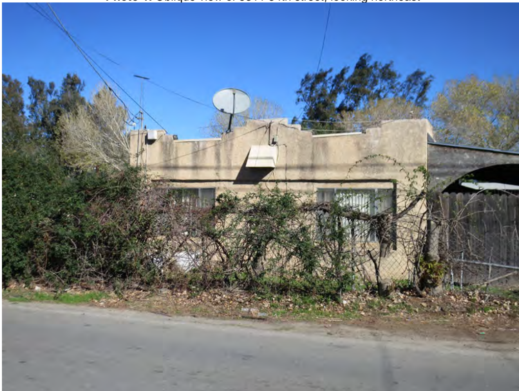
Photo 2. View of south façade of 5311 34th street, looking north
