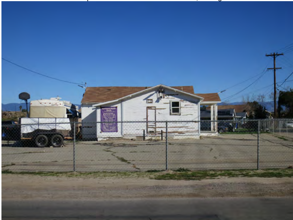
Photo 2. View of south façade of house at 5413 34th street., looking north
