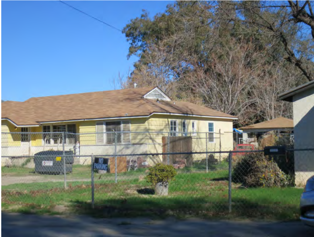
Photo 1. Oblique view of 5337 34th Street, looking northwest
