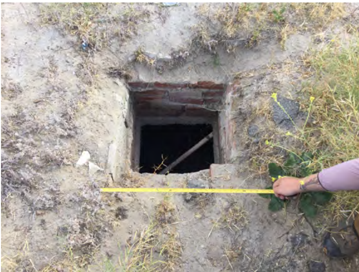
Figure 3. Cistern or other underground water feature.
