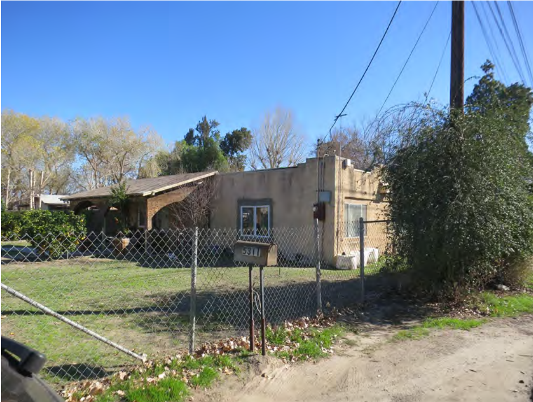
Photo 1. Oblique view of 5311 34th street, looking northeast
