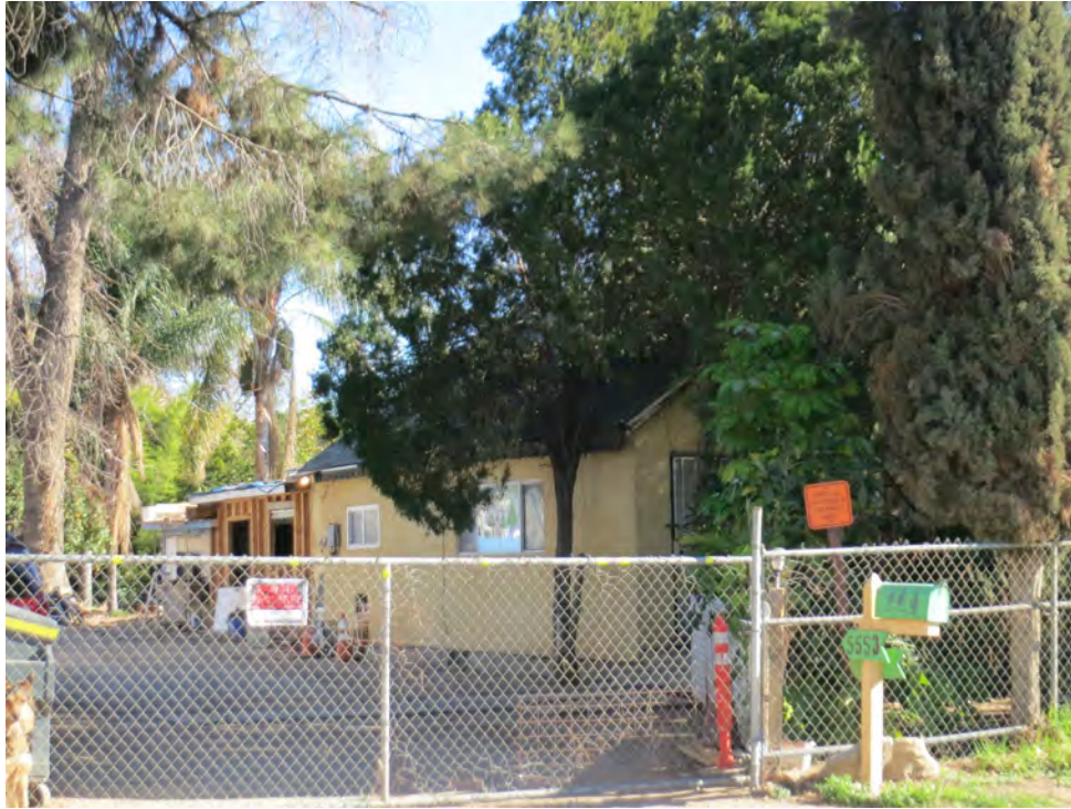
Photo 1. Oblique view of 5553 34th Street, looking northeast
