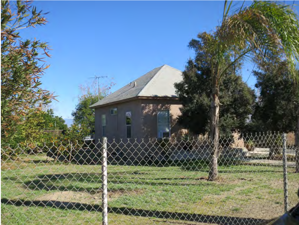
Photo 1. Oblique view of 5219 34th Street, looking northeast
