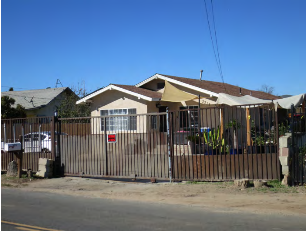
Photo 1. Oblique view of 3317 Wallace Street, looking southwest
