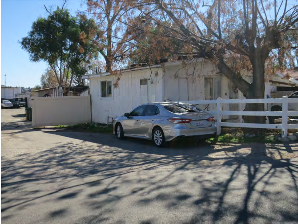
Photo 1. Oblique view of 3166 Wallace Street, looking south
