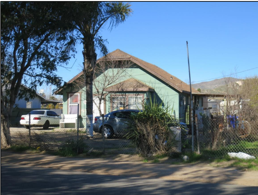
Figure 12. West façade of 3343 Wallace Street, looking southwest.
