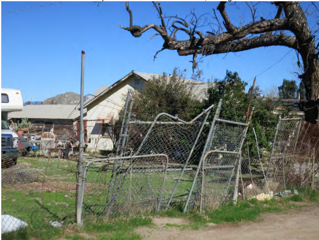
Photo 2. Oblique view of 3333 Wallace Street, looking southwest
