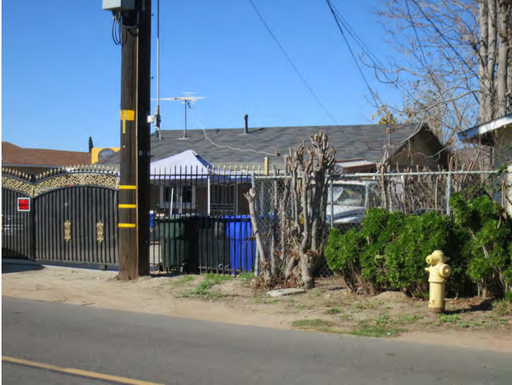
Photo 1. Oblique view of 3309 Wallace Street, looking southwest
