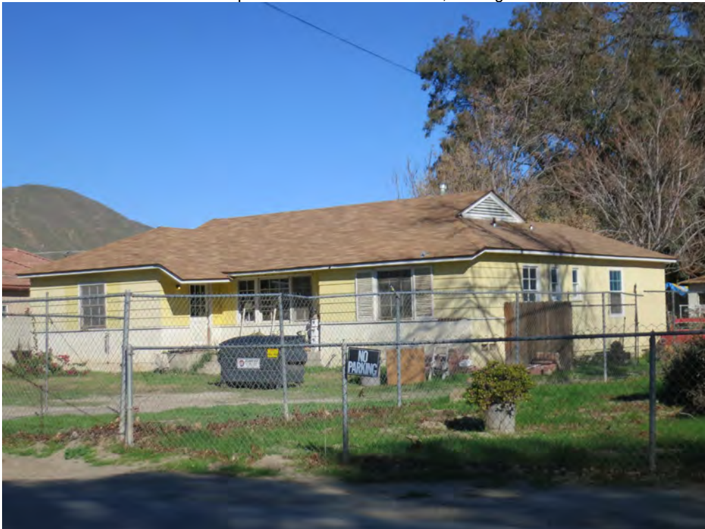
Photo 2. Oblique view of 5337 34th Street, looking northwest
