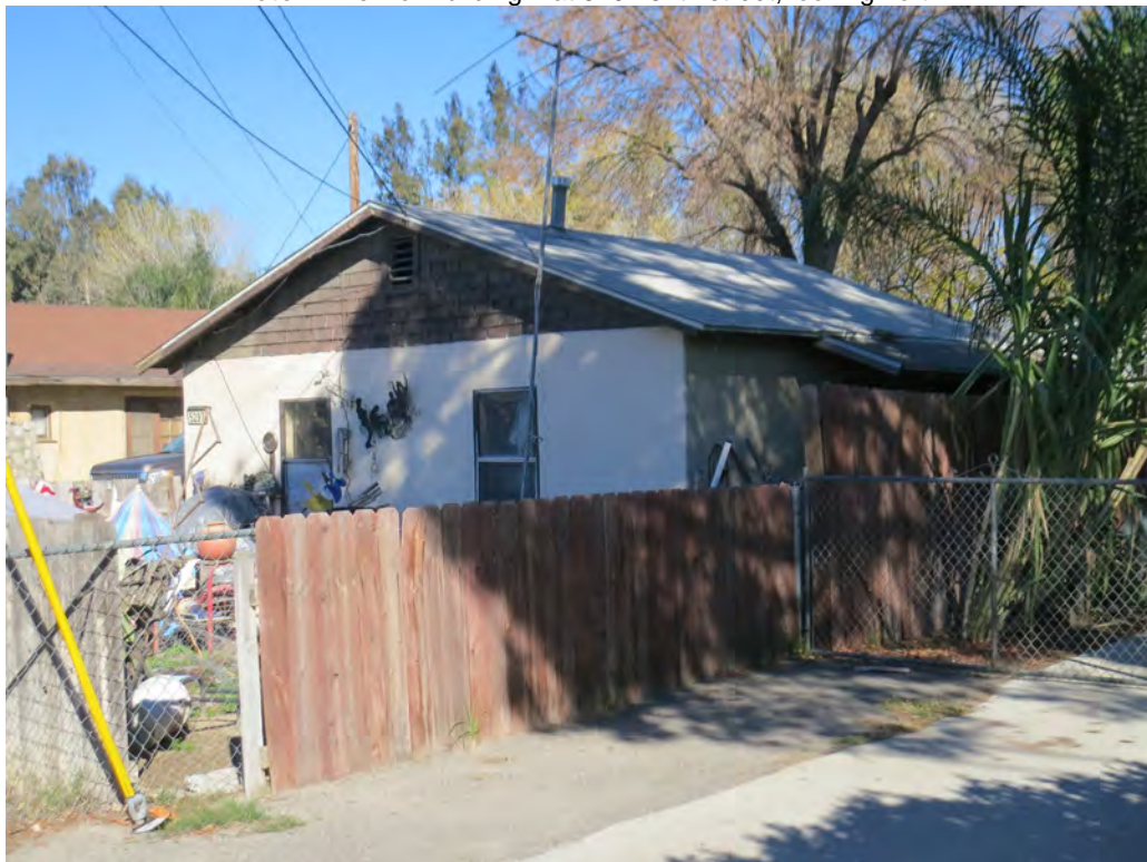
Photo 2. Oblique view of Building 1 at 5297 34th street, looking northwest
