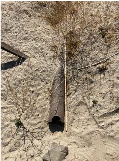
Figure 2. Buried pipe within the trench
