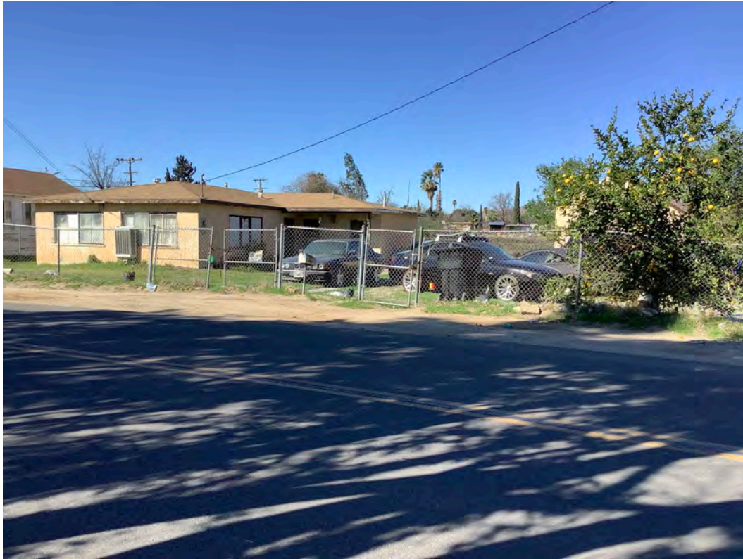
Photo 1. Oblique view of 3377 Wallace Street, looking southwest
