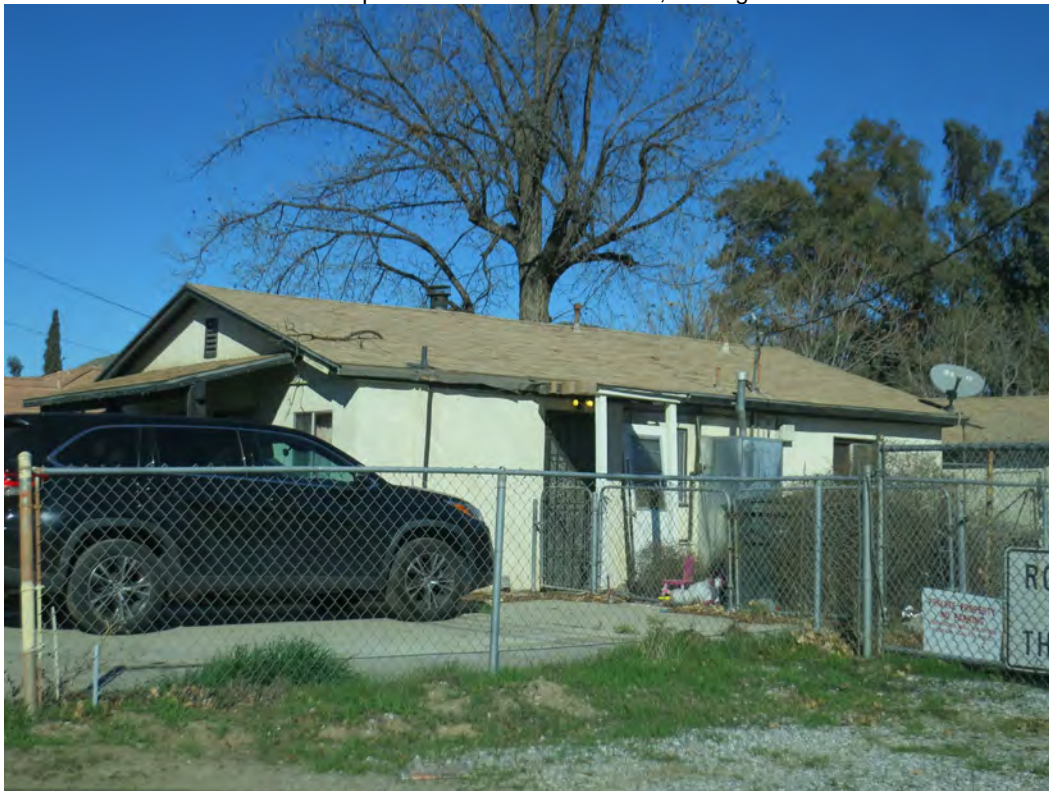
Photo 2. Oblique view of 5325 34th Street, looking northwest
