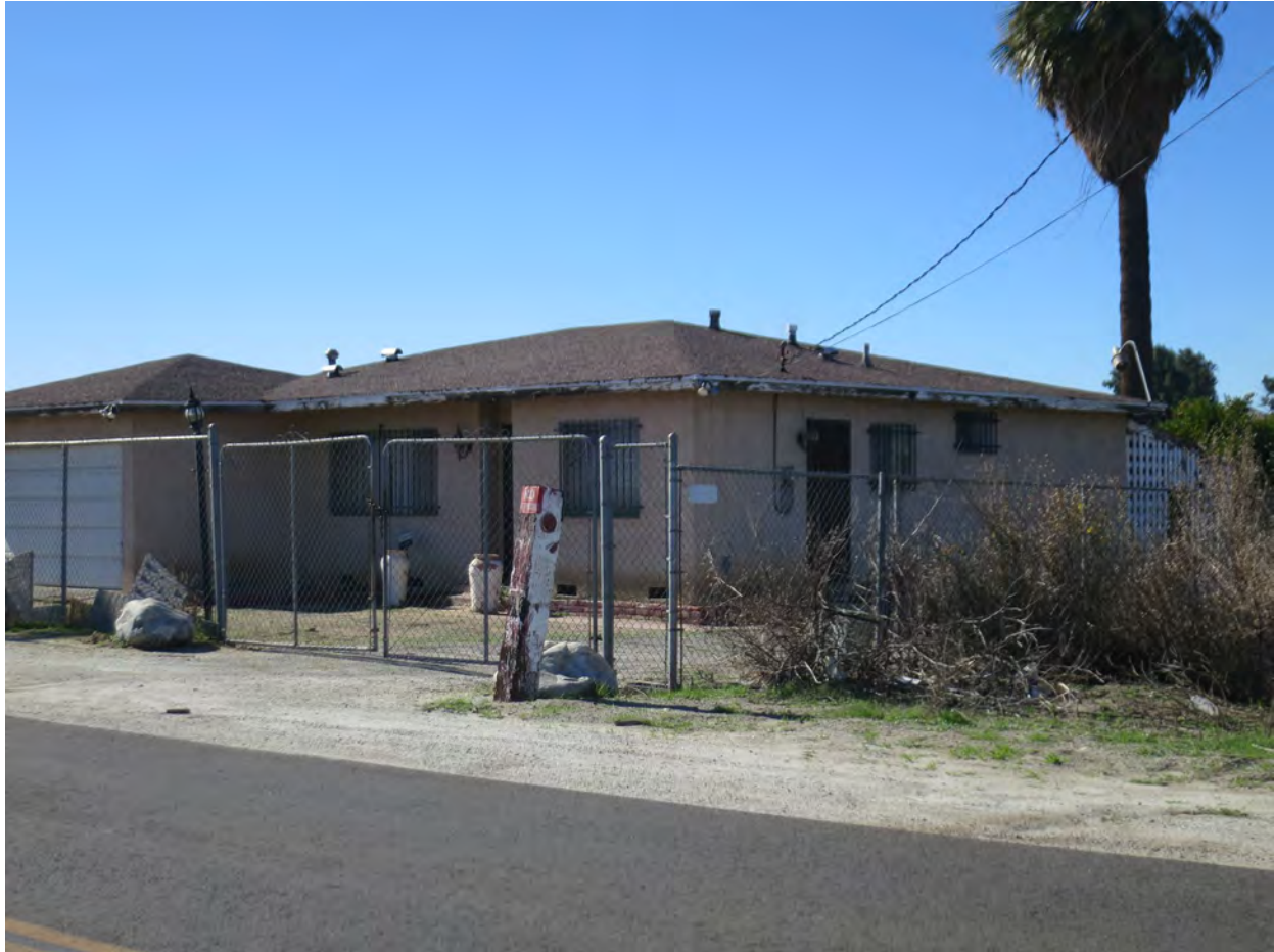
Photo 1. Oblique view of 2861 Wallace Street, looking southwest
