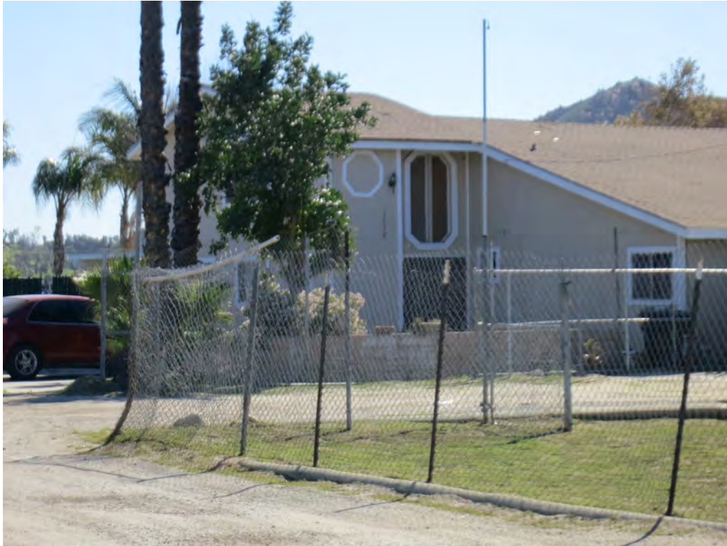
Photo 1. Detail view of 3150 Wallace Street, looking southeast
