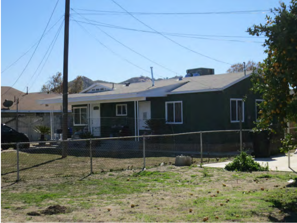
Photo 1. Detail view of 3156 Wallace Street looking southeast
