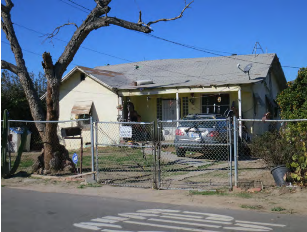
Photo 1. Oblique view of 3333 Wallace Street, looking southwest
