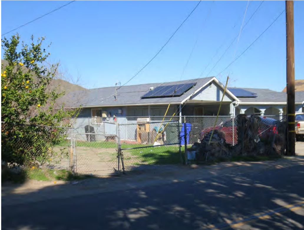
Photo 1. Oblique view of 3345 Wallace Street, looking northwest
