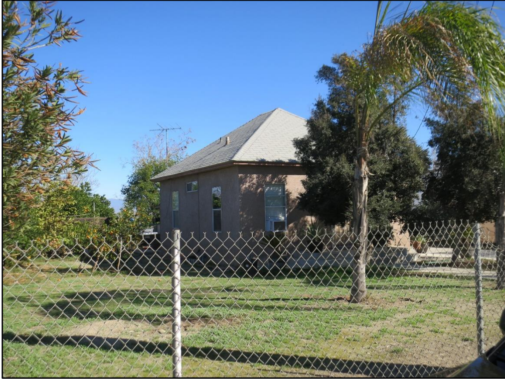
Figure 9. View of 529 34 th Street, looking northeast.
