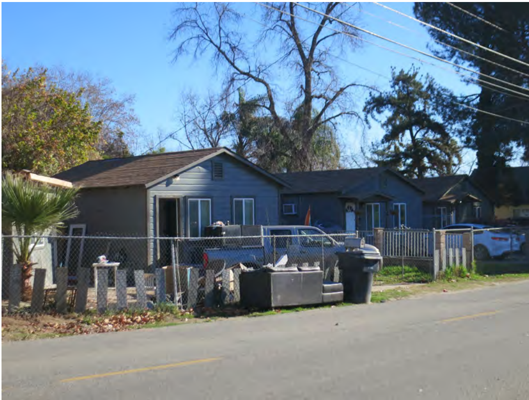
Photo 1. Oblique view of 5557, 5565, and 5567 34th Street, looking northeast
