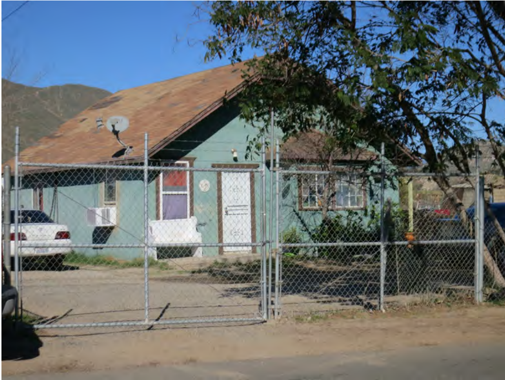
Photo 1. Oblique view of 3343 Wallace Street, looking northwest
