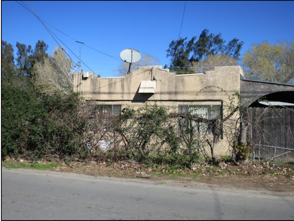
Figure 13. View of south façade of 5311 34 th Street, looking north.
