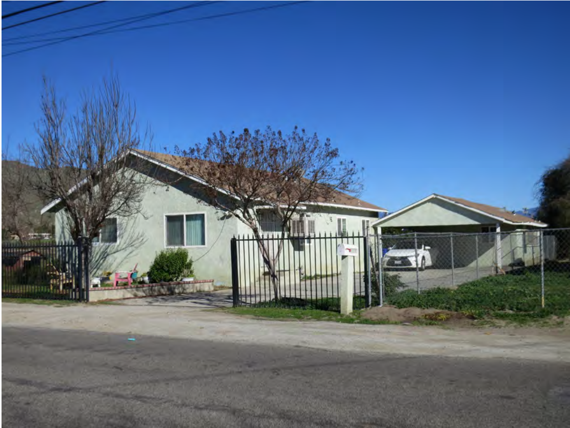
Photo 1. Oblique view of 5421 34th Street, looking northeast
