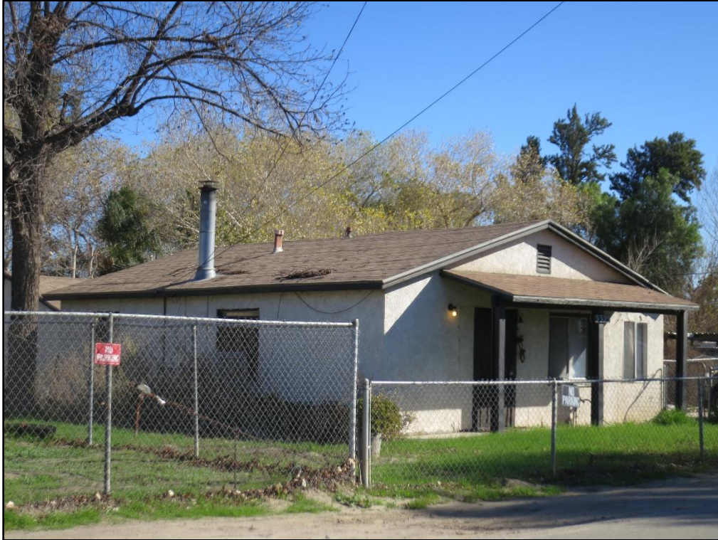
Figure 15. Oblique view of 5325 34 th Street, looking north.
