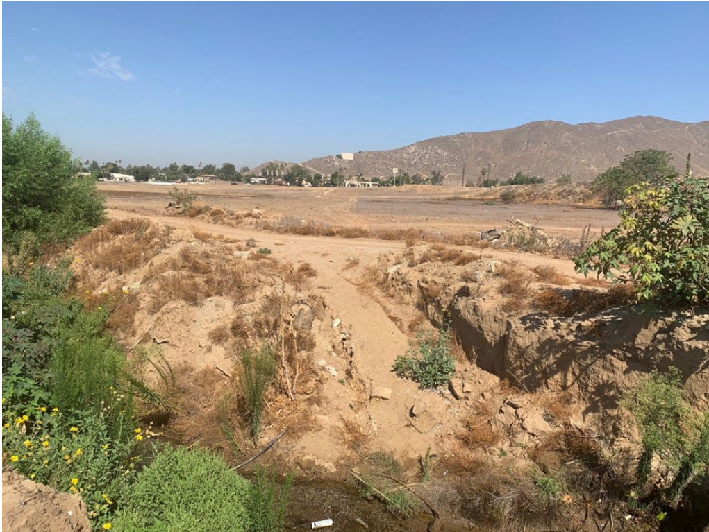
Photograph 2: Looking northwest across the earthen portion of the Jurupa Ditch. Note the heavy presence of clay soils along the banks. The Jurupa Ditch has been in existence for 140 years.
