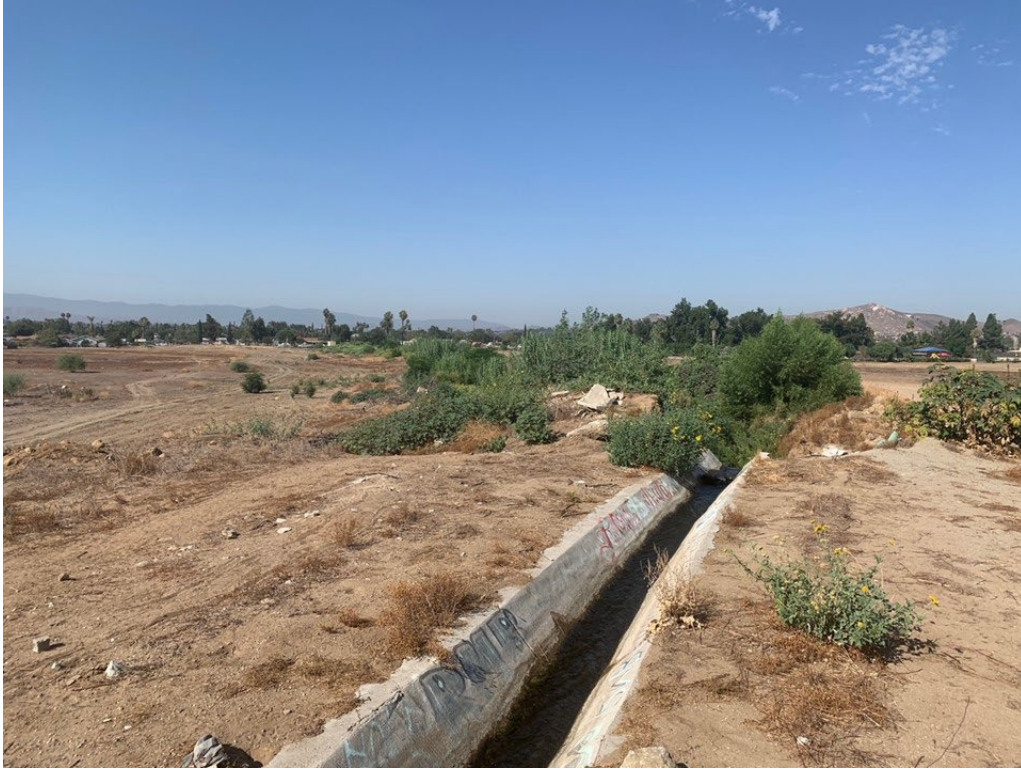
Photograph 1: Looking southwest from the inside the northern boundary at the top of the Jurupa Ditch where water from the Santa Ana River is released from concrete channel into an earthen channel. Delhi Sand soils are mapped on either side for the channel extending out 200 yards on each side of the channel.
