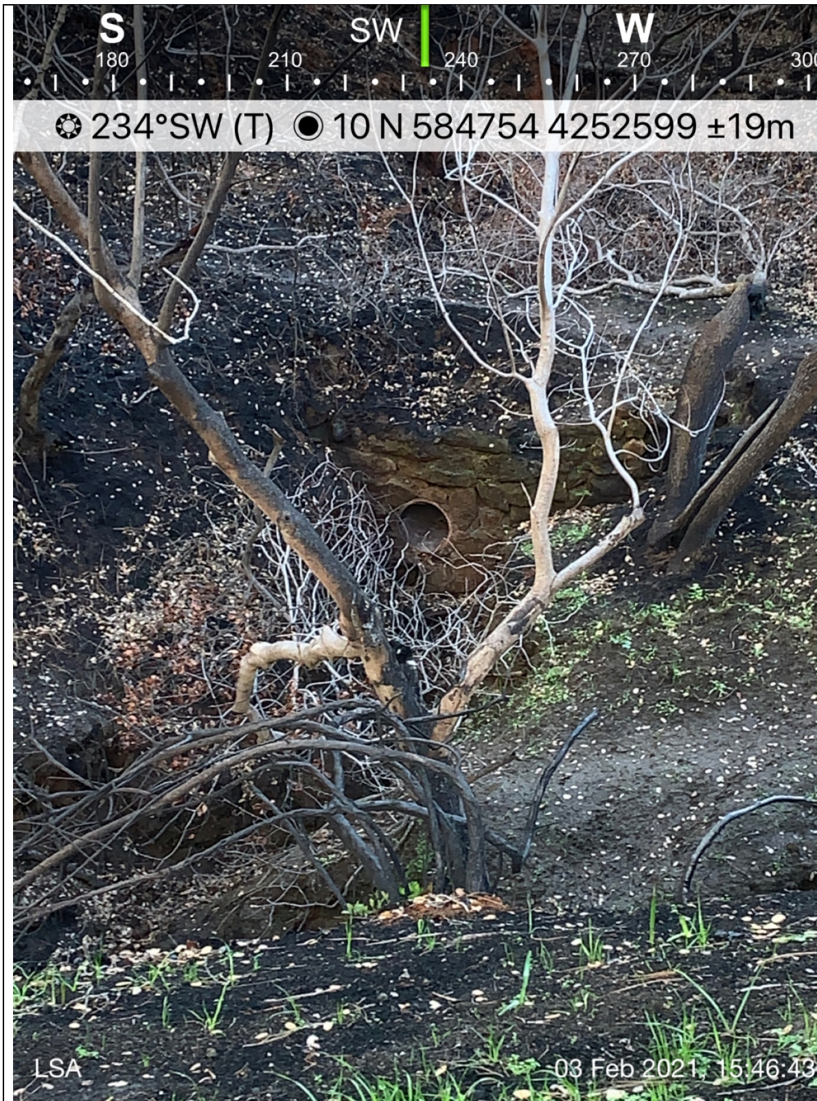
Drainage culvert and stonework
