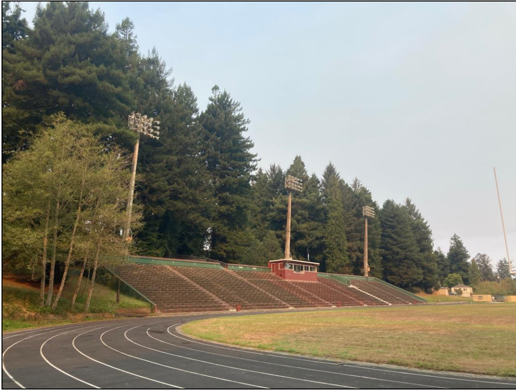
Figure 12. Albee Stadium Lighting (West)
