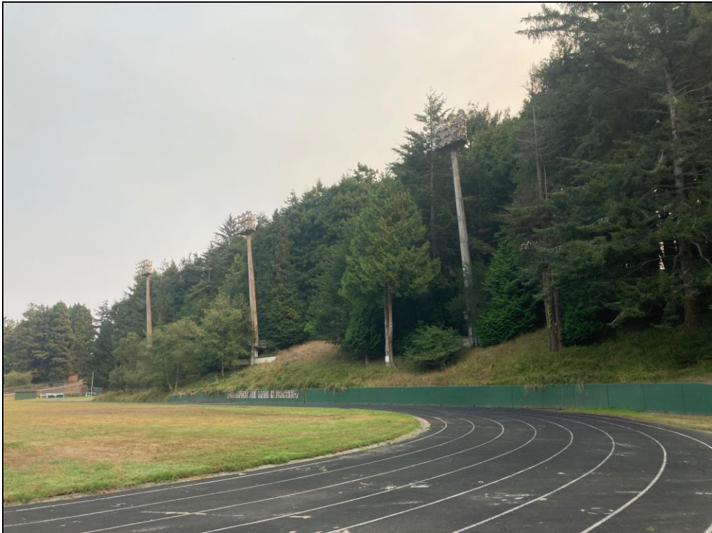
Figure 13. Albee Stadium Lighting (East)
