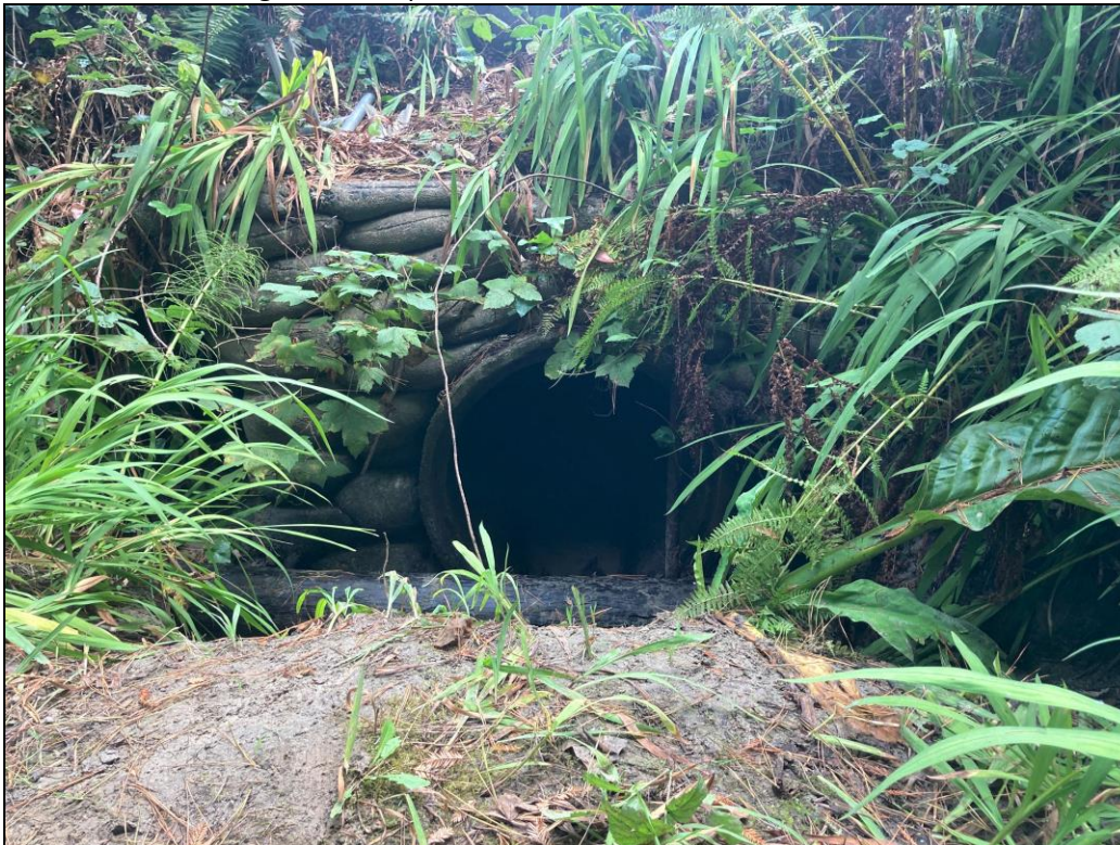
Figure 16. Cooper Creek Storm Drain Inlet and Headwall
