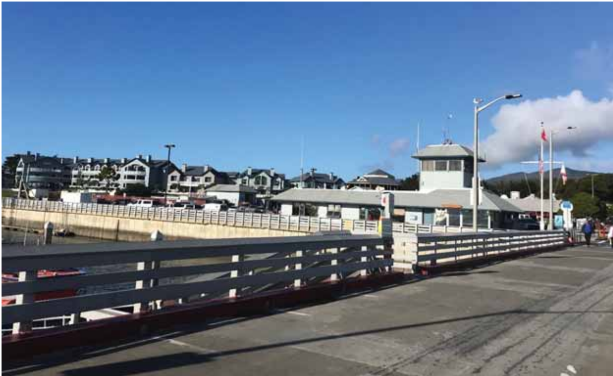
Photograph 8. View of Johnson Pier, the Pillar Point Harbor Office Building, and surrounding hotel, restaurants, and retail buildings, facing northwest.
