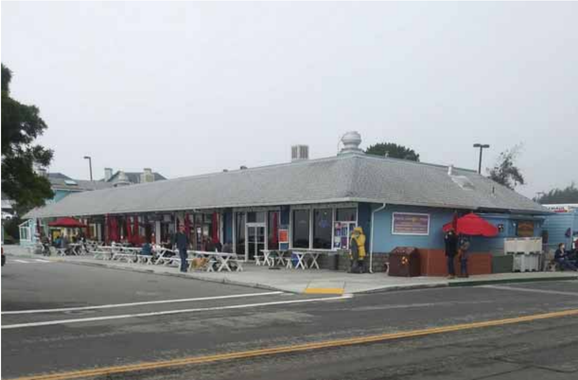
Figure 5 Commercial Building, South and East Elevations, Facing Northwest
