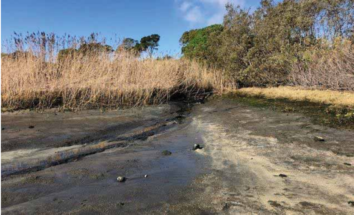
Photograph 9. View of the outlet of the culverted drainage flowing into Pillar Point Harbor from Pillar Point Harbor Boulevard, facing north. Common reeds are growing to the left of the drainage, while arroyo willows are growing to the right.
