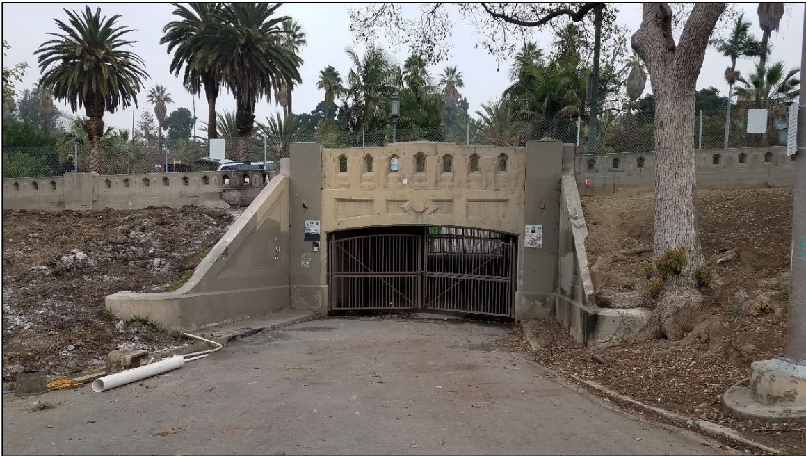
Figure 11. View of the Wilshire Boulevard underpass.
