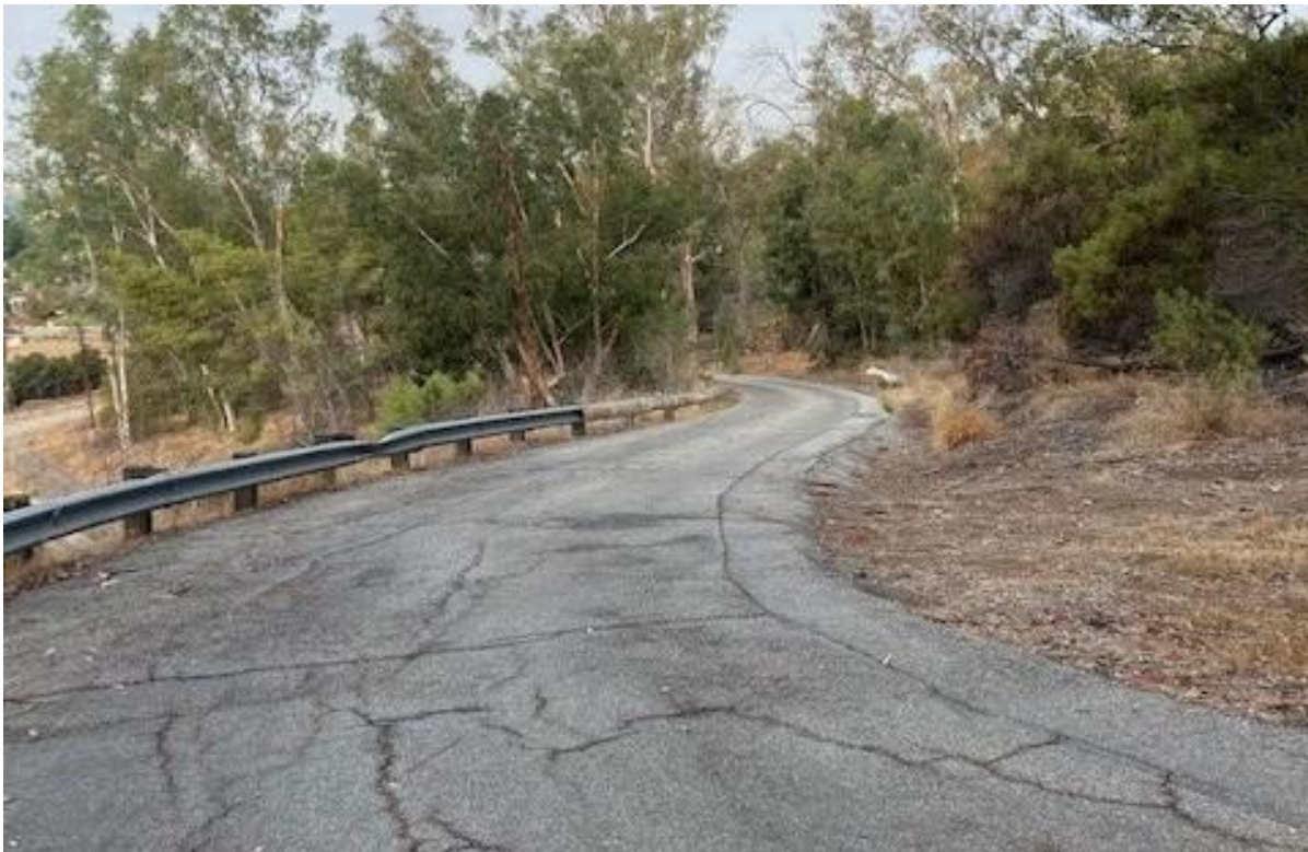
Figure 9 Access Road Near Reservoirs, Facing Southwest, August 2021
