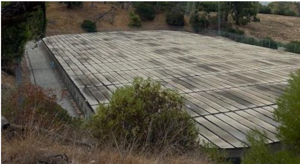
Figure 5 Reservoir No. 9 Surface, View Southeast
