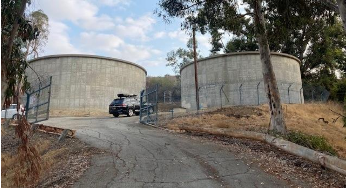
Figure 4 Murphy Reservoirs, Reservoir 11 (Left) and Reservoir 10 (Right), View North
