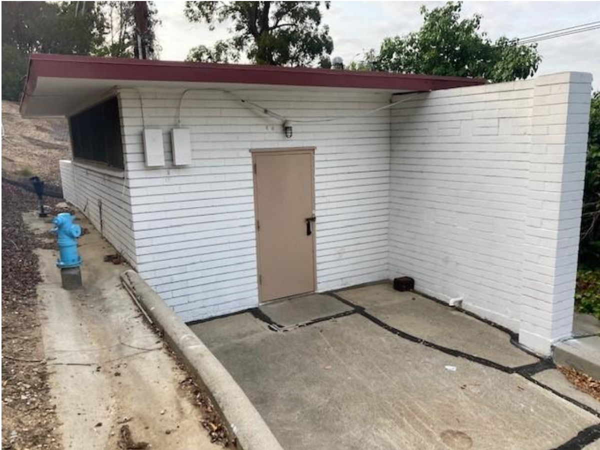
Figure 6 Primary Elevation of Murphy Booster Pump House, view southeast
