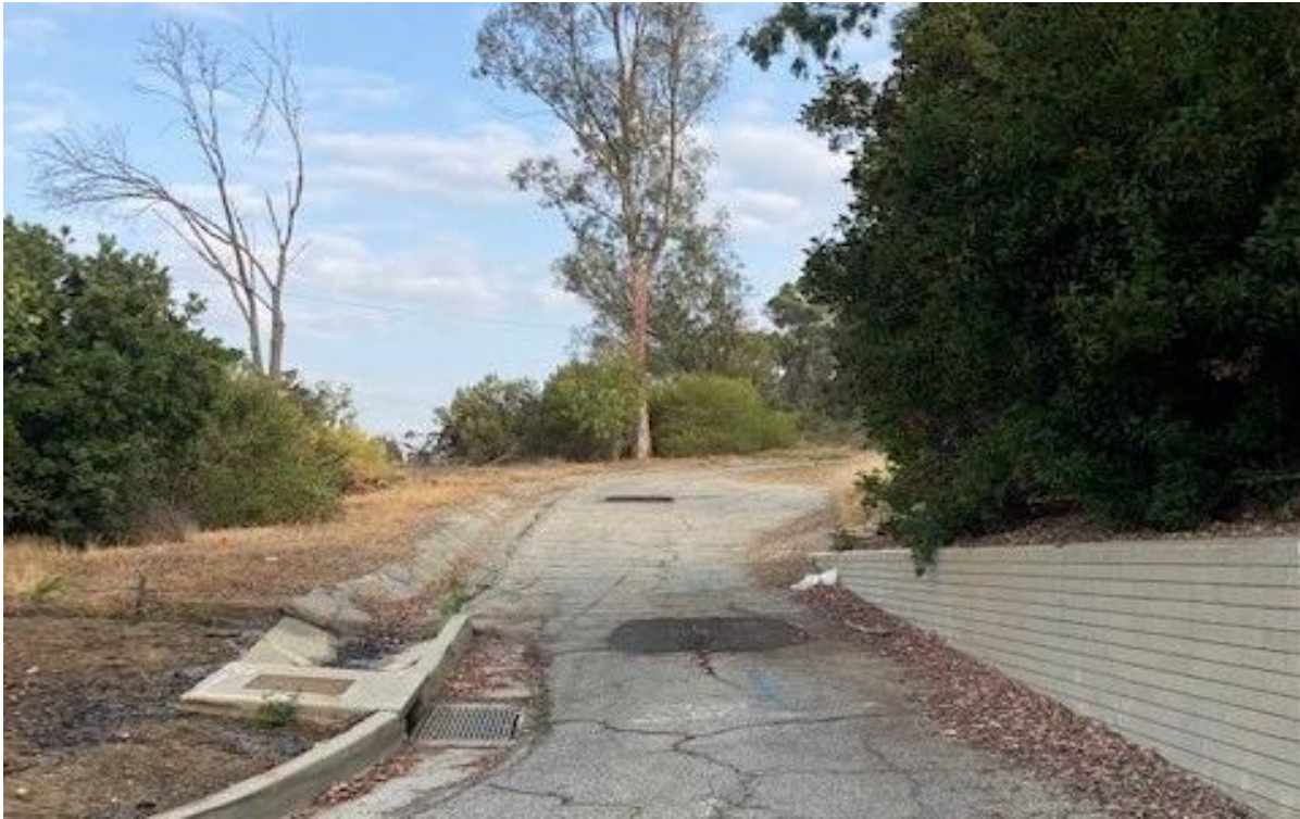
Figure 8 Access Road Near Entrance, Facing Northwest, August 2021
