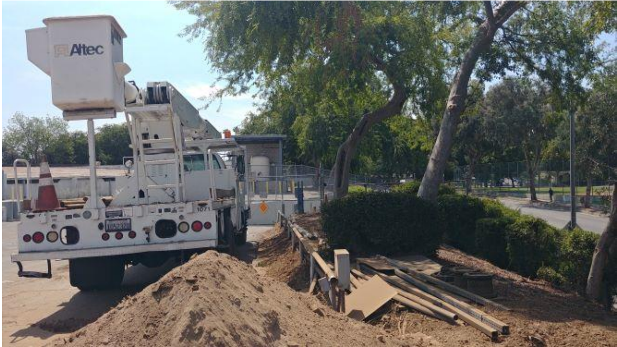
50. Trees #16-18 (R-L). Note lean on #17 and decay cavity on #18.
