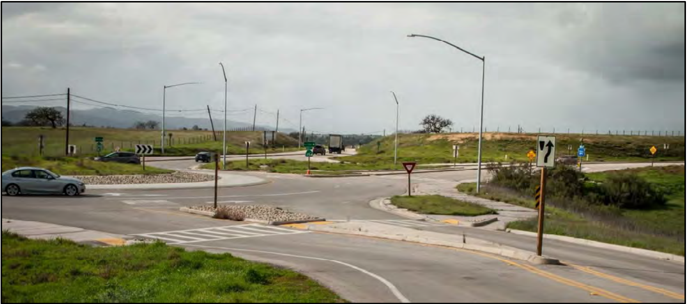
Pedestrian Crosswalk at SR 154/SR 246 Roundabout
