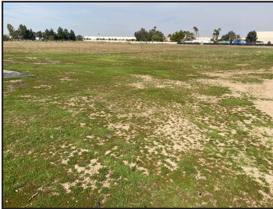
PHOTOGRAPH 1 - Northwest view of Project Site from southeast corner adjacent to East Nance Street.
