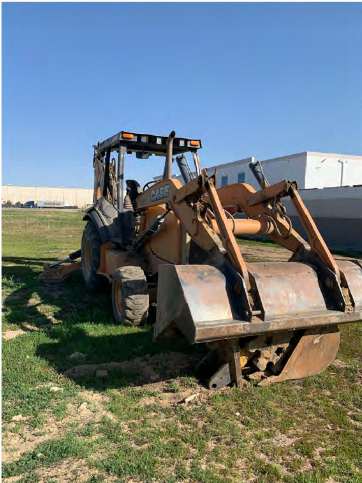
Backhoe Staged at the Site
