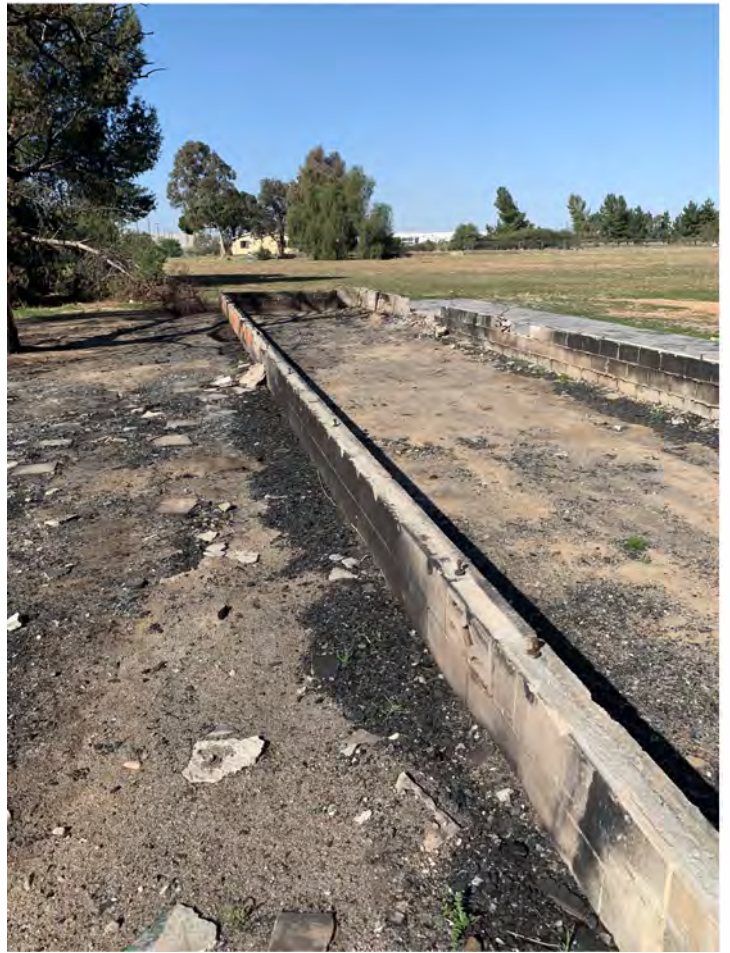
Footprint of Former Structure
