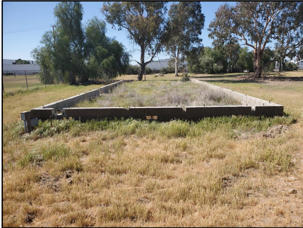
Plate 3: Overview of a modern foundation, facing south.
