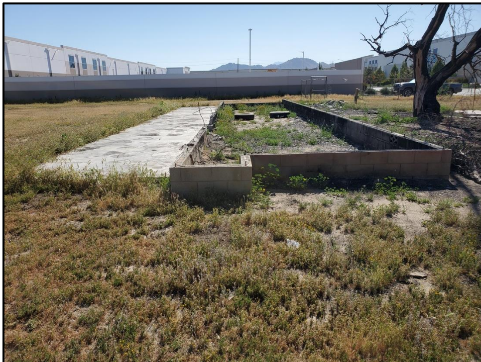
Plate 4: Overview of a modern foundation, facing south.
