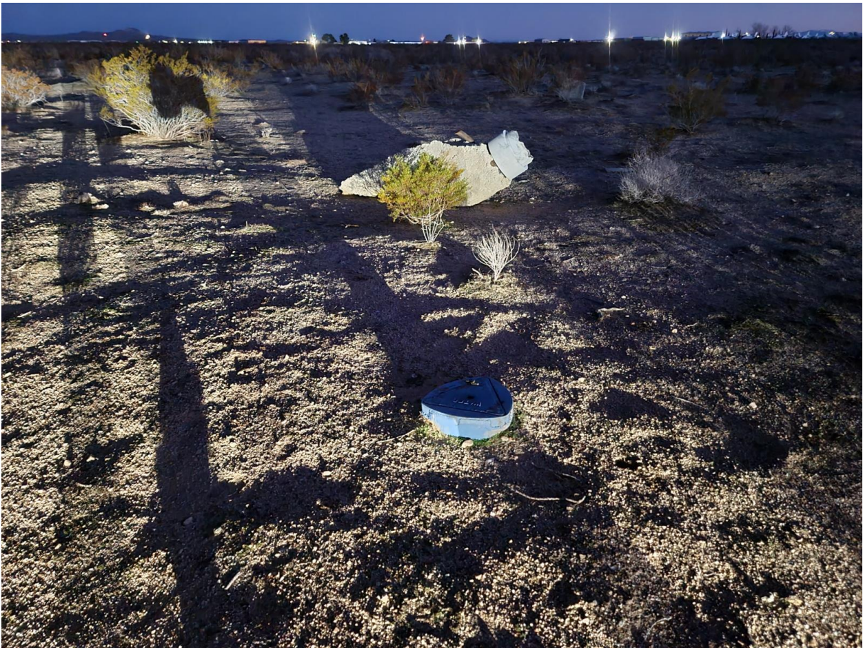
WATER VALVE NORTHEAST OF SITE ABOUT 1500 FEET AND ALONG SECTION LINE
