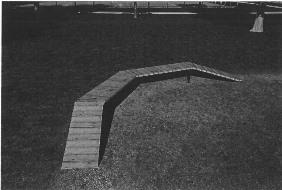
INTERMEDIATE WOODEN RAMP, 18"-24" WIDE, 90 DEGREE TURN
