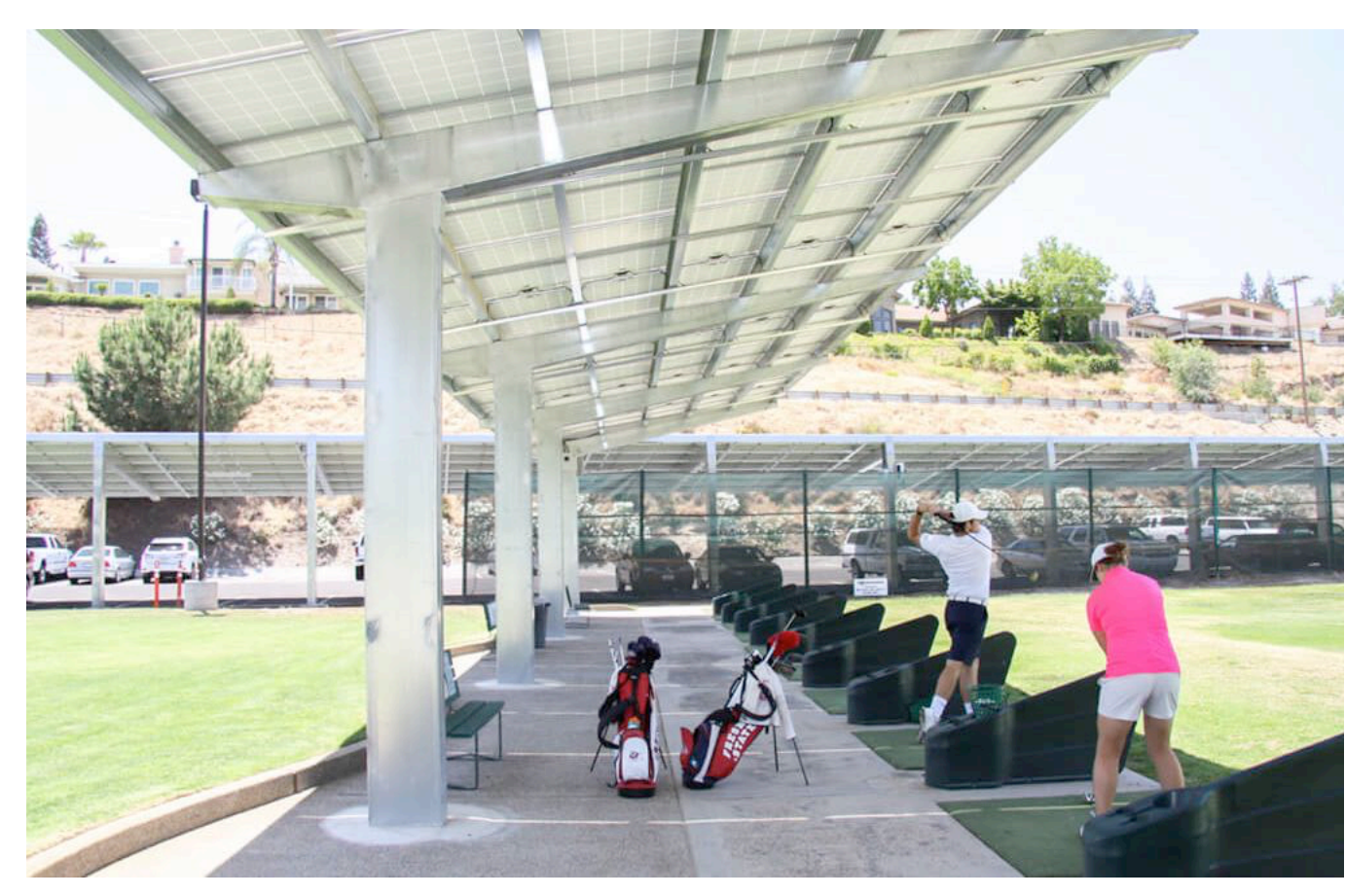
3 A3.0 EXAMPLE OF PROPOSED PREFABRICATED, GALVANIZED STEEL WALKWAY SHADE COVER W/ PV PANELS (BY BAJA CARPORT OR APPROVED EQUAL)
