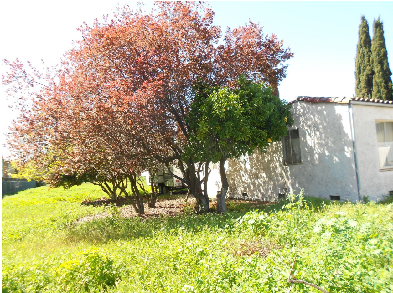
Photograph 3 101 Jackson Ave. Main house View: south side facade (facing northwest) Date: 3/2018
