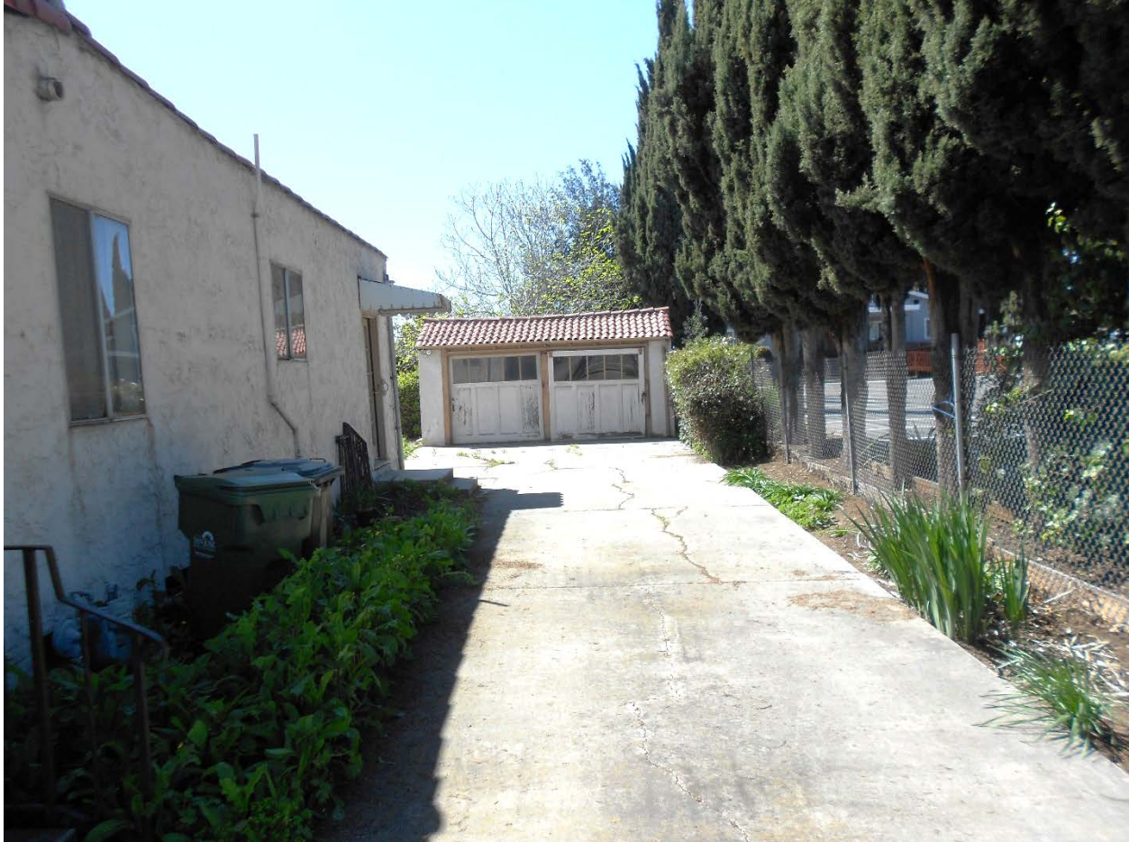
Photograph 4 101 Jackson Ave. Main house View: North side facade and garage (facing west) Date: 3/2018
