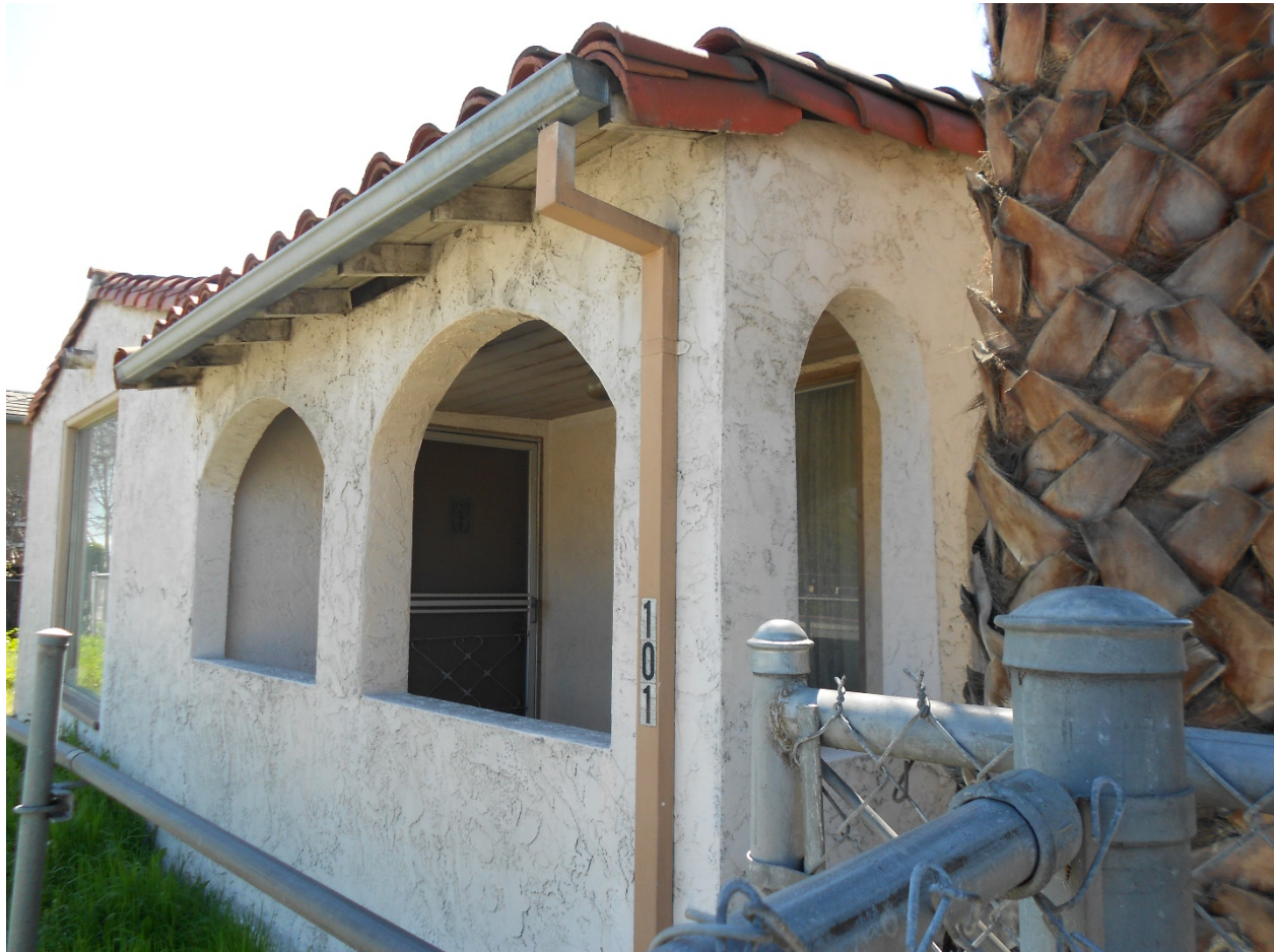
Photograph 2 101 Jackson Ave. Main house View: Front facade (facing south) Date: 3/2018
