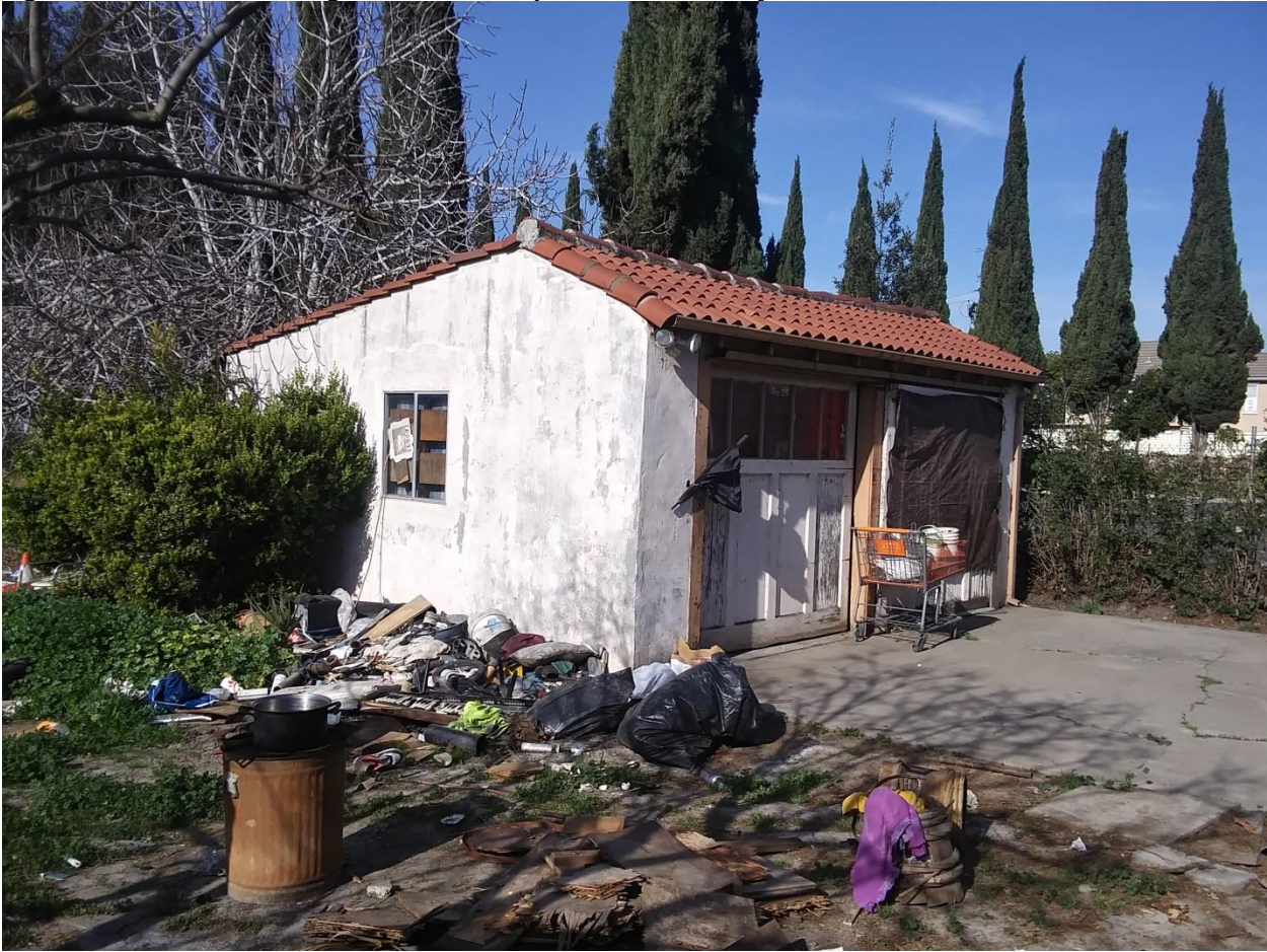
Figure 4. Detached Garage and Driveway Structure on Project Site
