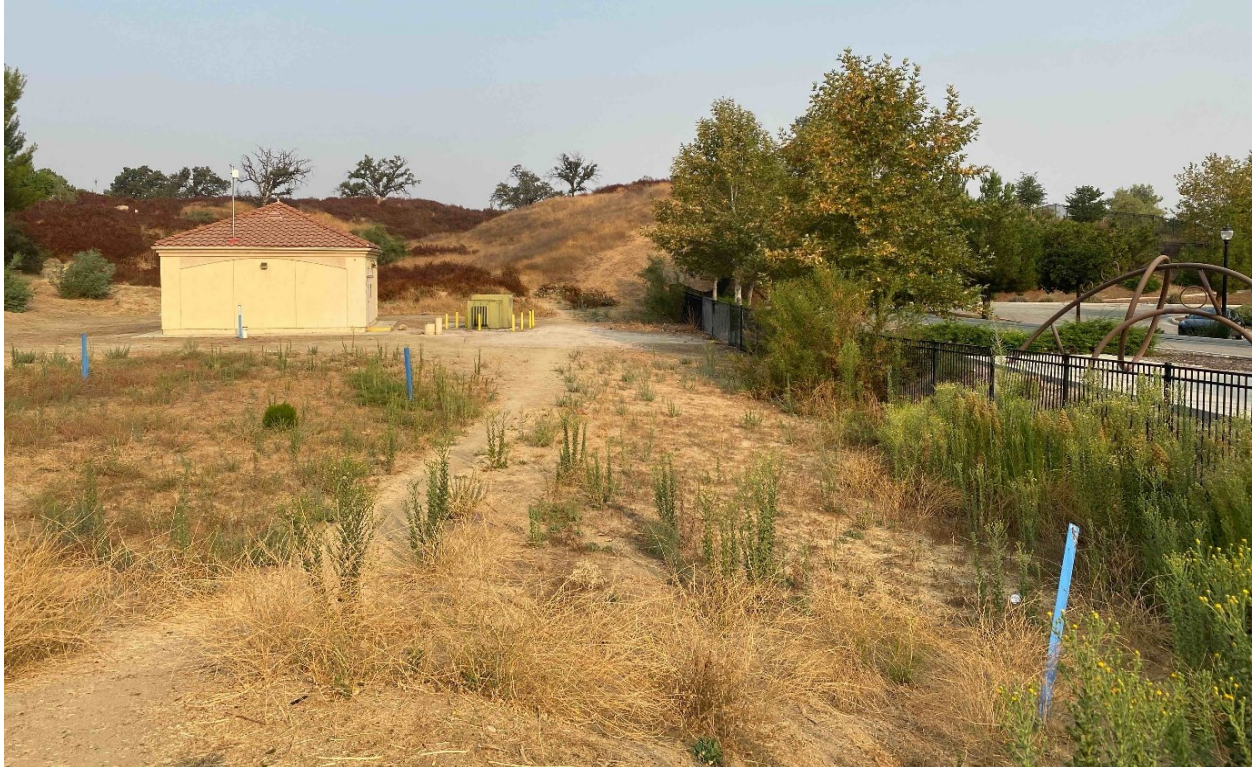
Photograph 1. View of existing Well 205 facility, facing northwest. September 14, 2020.
