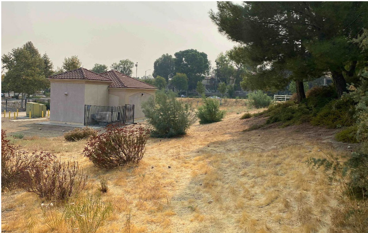
Photograph 4. View of existing Well 205 building, taken from western portion of site facing east towards Valencia Boulevard.
