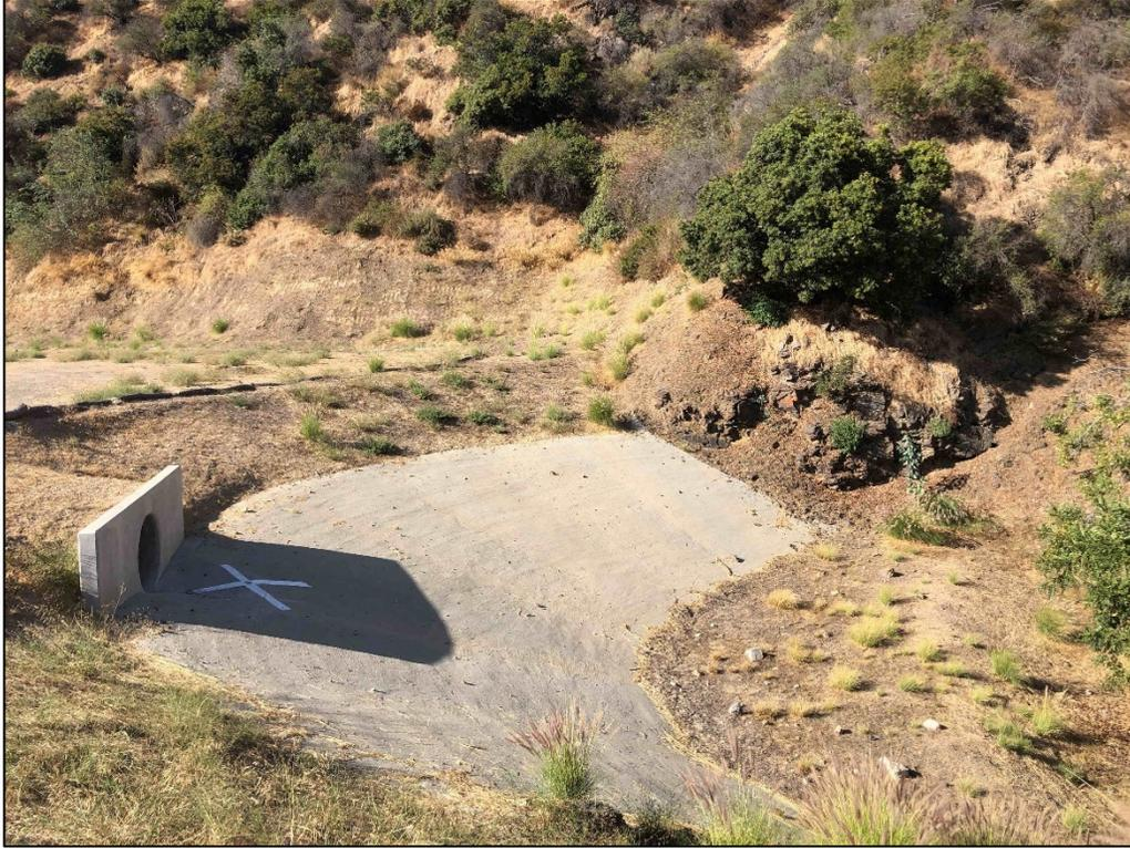
Photo 9. Concrete Drainage Basin with Headwall Adjacent to Oak Parking Lot B, View Facing Southwest
