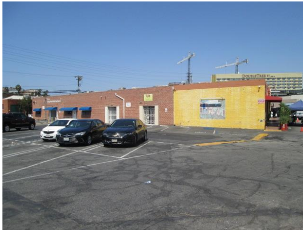
5. 6520 Arizona Avenue building.
