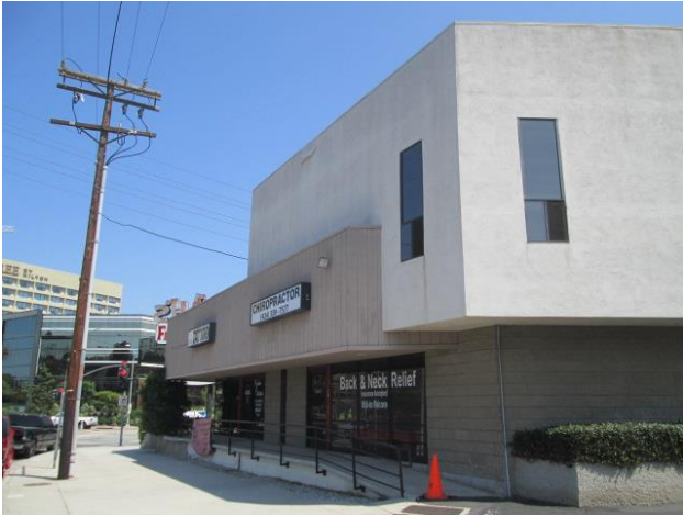
1. Northwest portion of the 6501 S. Sepulveda building.
