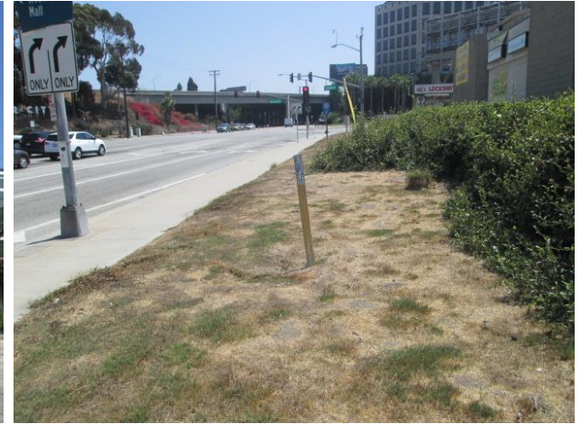
21. Northern adjoining landscaped areas. Note petroleum pipeline placards.
