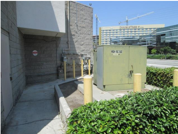
10. Electrical transformer.
