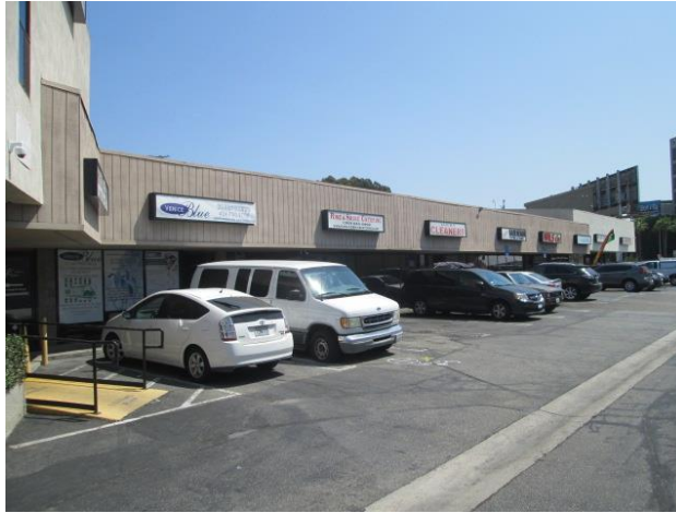
2. 6501 S. Sepulveda building.
