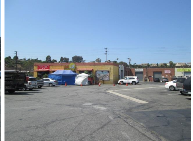
3. 6520 Arizona Avenue building.
