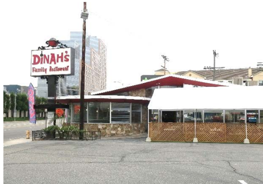
View south of the north (primary) façade, east end and 1971 pylon sign ("A" on Map 3) (ARG, 2020).
