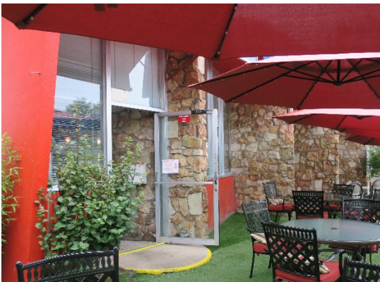
View northwest of the east façade (ARG, 2020).
