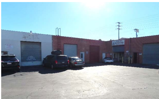
View southwest of the north façade (ARG, 2021).
