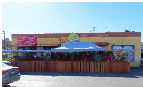
View west of the east façade. Note altered fenestration/window openings (ARG, 2021).
