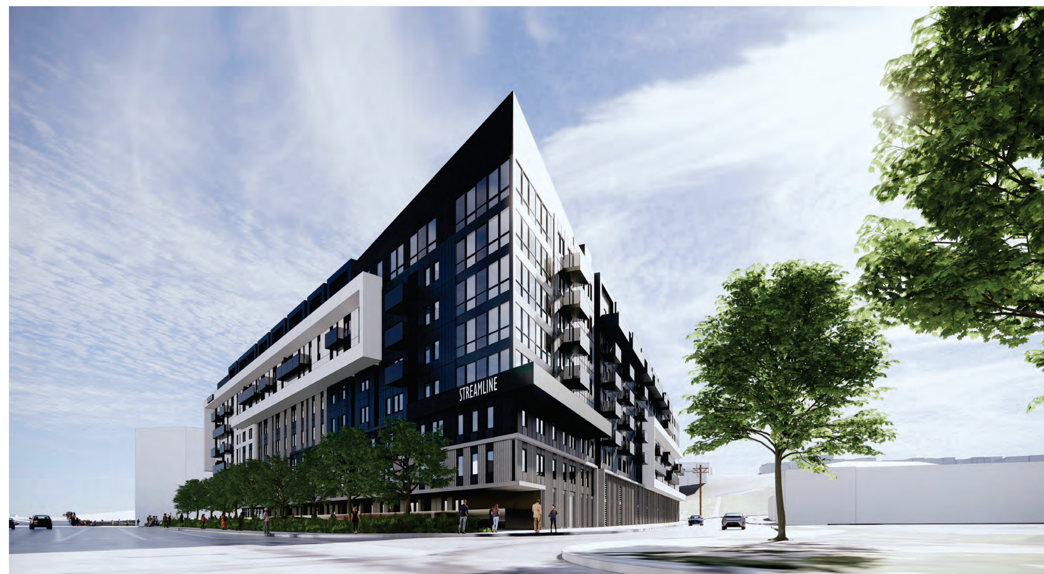
CORNER OF CENTINELA AND ARIZONA
