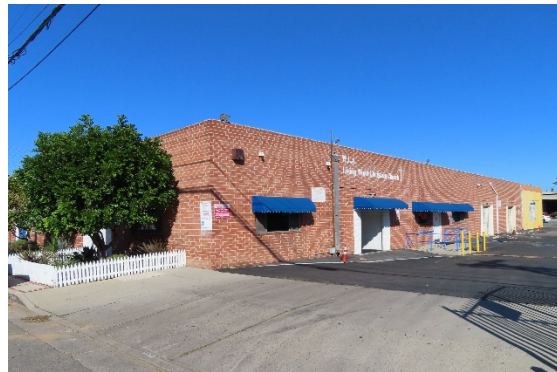
View northeast of the south and west façades (ARG, 2021).
