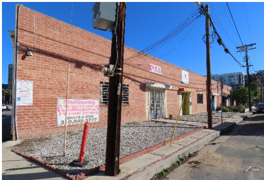
View southeast of the west façade, along Arizona Avenue (ARG, 2021).
