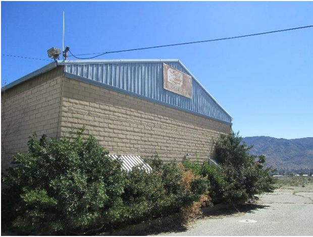
25. West side of the Site building.
