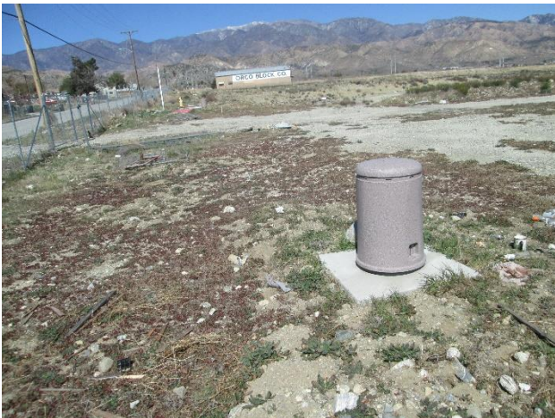
28. Utility feature in the southwest portion of the Site.
