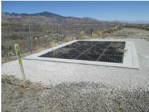
23. Gas pipeline vault.
