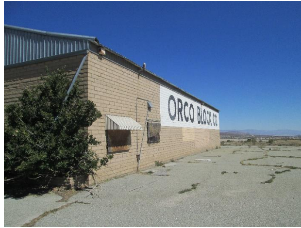
26. South side of the Site building.
