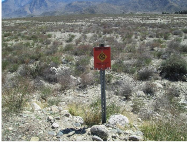
20. Fiber optic utility placard.
