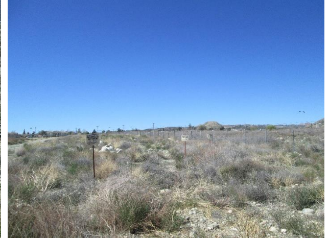
21. High pressure gas pipeline placards.
