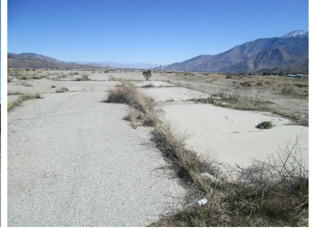
9. Typical paving in the northwestern portion of the Site.
