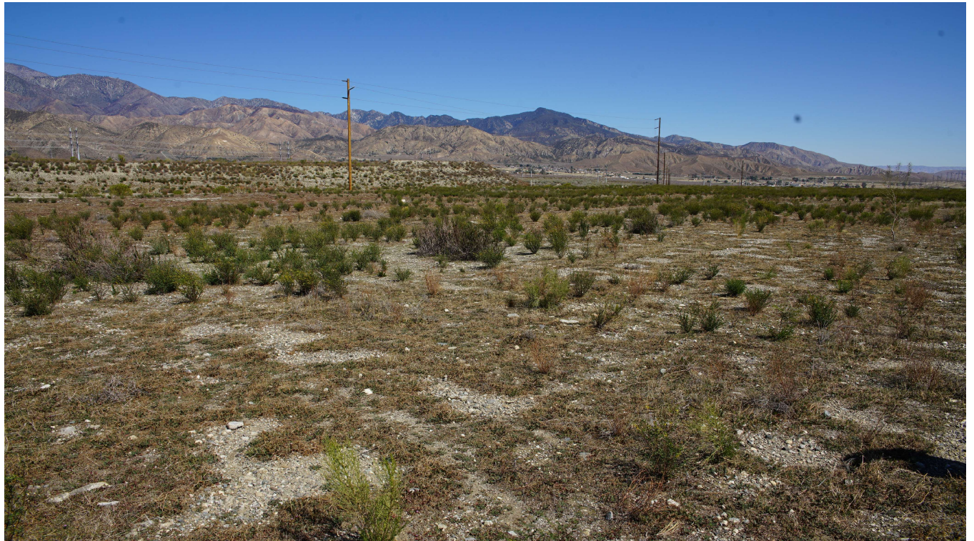
Photograph 2 Looking North over Center of Property - Graded pads, slopes and roads. Hydroseeded
