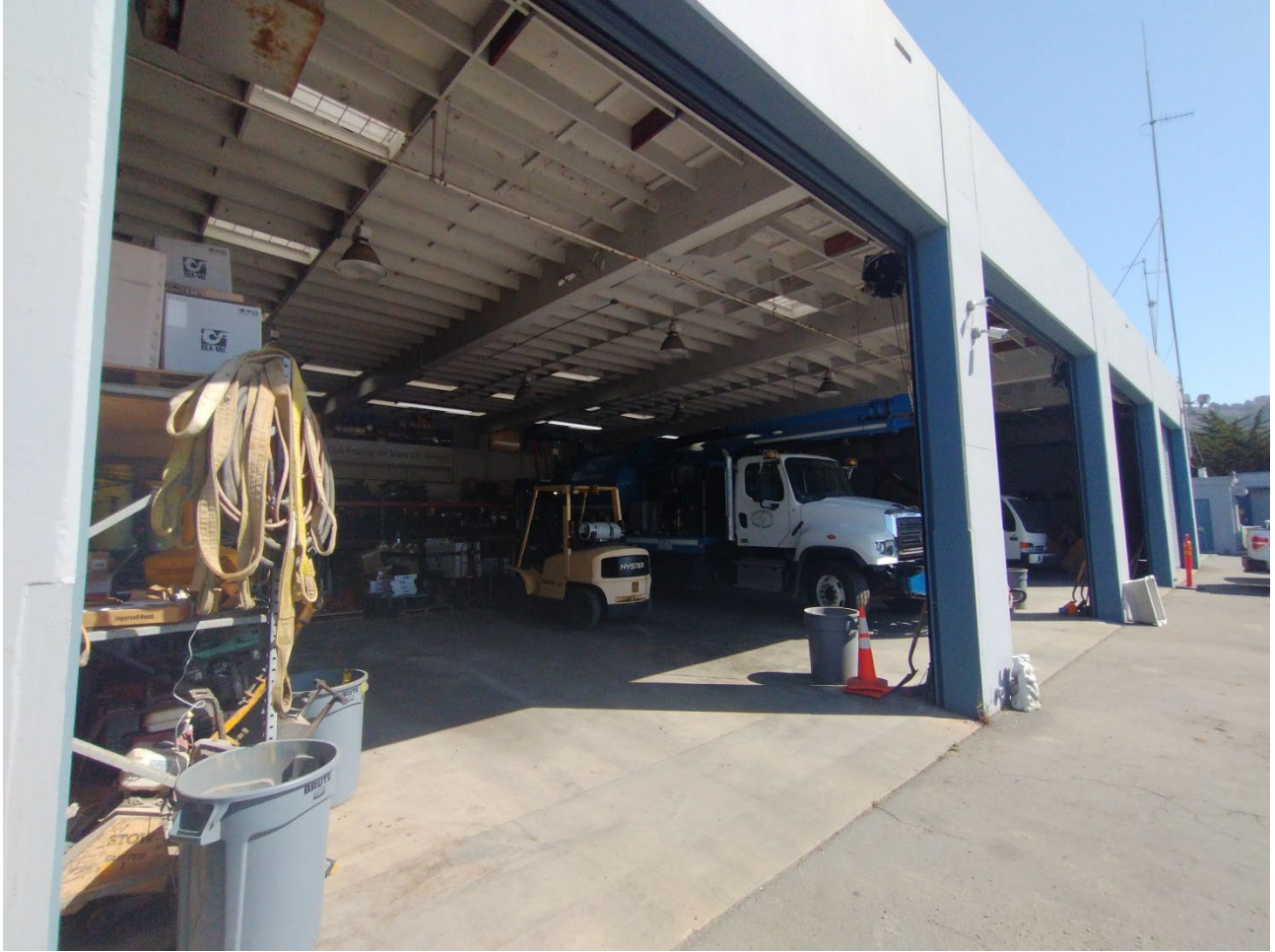
Figure 15 The four garage bays of Building No. 2/Maintenance No. 2, as viewed to the northeast. Note the skylights and unpainted bracing joist blocks from the 1998 seismic retrofit, visible just above the interior of the garage-door lintels. Photograph by Yarbrough Architectural Resources, Sept. 15, 2021.
