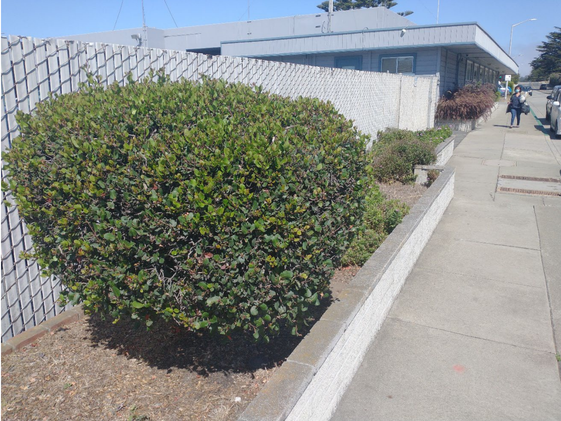
C-1. Concrete masonry unit planting boxes fronting Francisco Boulevard with security fence and Building No. 1 in the background, view to the northwest. Photograph by Yarbrough Architectural Resources, Sept. 15, 2021.
