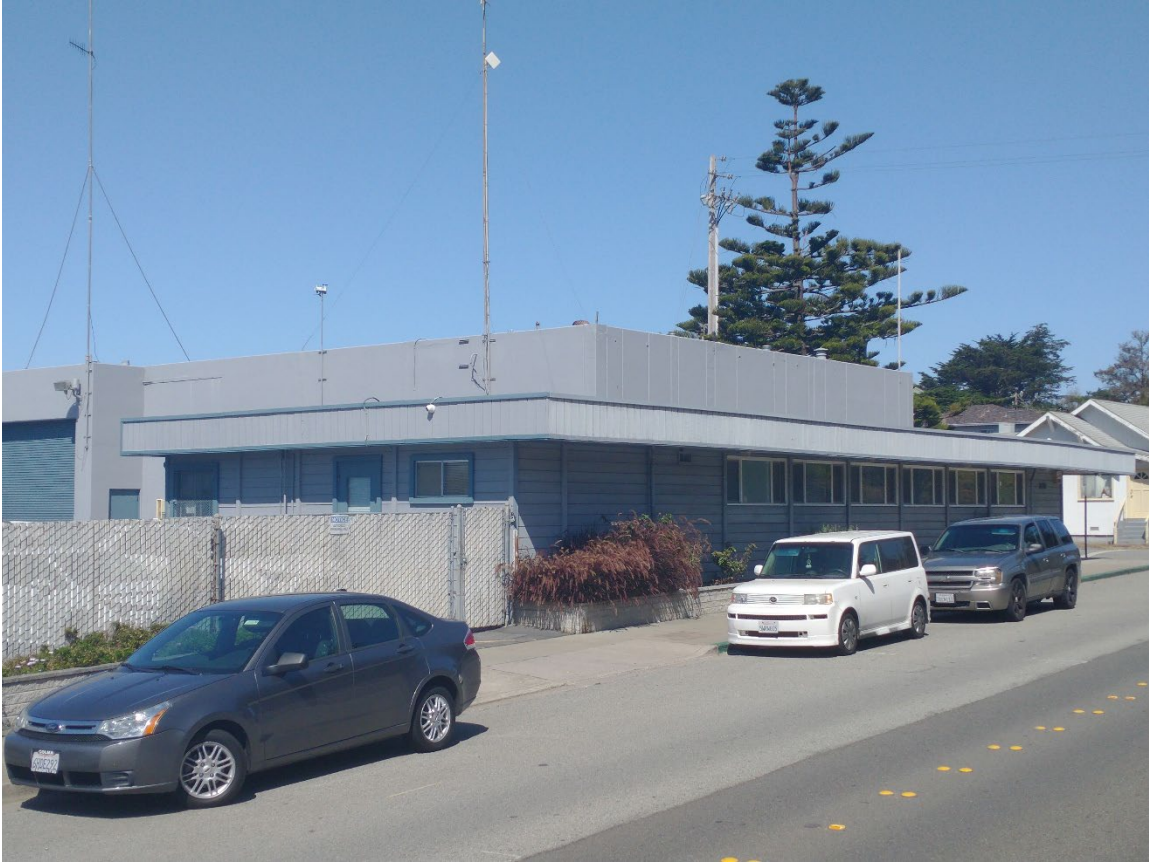
C-4. Building No. 1, Francisco Boulevard and the Administrative Building in the foreground with the taller Maintenance No. 1 portion behind. Communication antennae are secured to the building roof. Photograph by Yarbrough Architectural Resources, Sept. 15, 2021.
