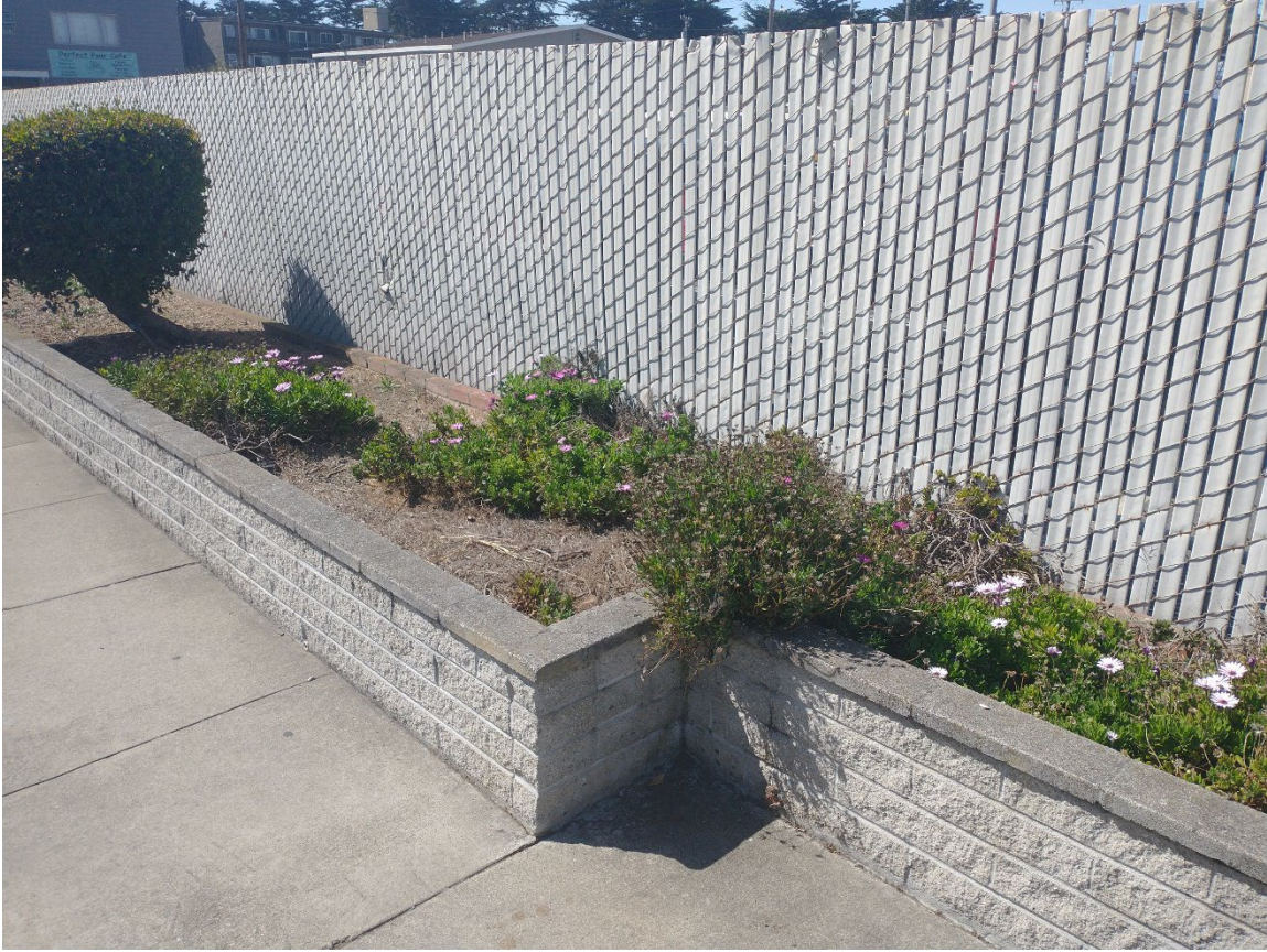
C-2. Concrete masonry unit landscape box fronting Francisco Boulevard Photograph by Yarbrough Architectural Resources, Sept. 15, 2021.
