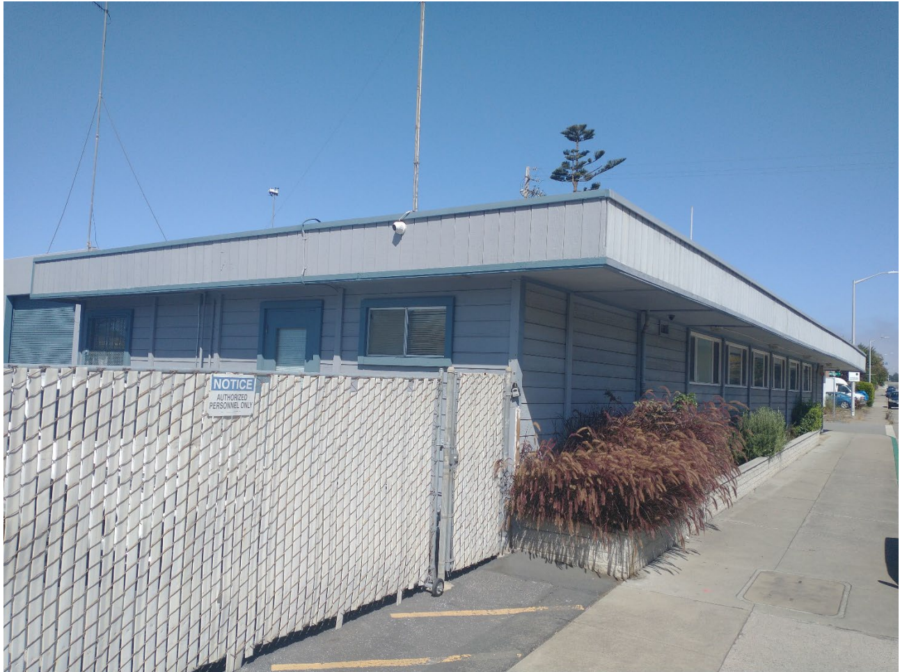
Figure 11 Administrative Building viewed to the north-northwest showing wood or composite wood horizontal clapboards on walls and vertical boards on thick, projecting cornice from 1979 remodel. Photograph by Yarbrough Architectural Resources, Sept. 15, 2021.
