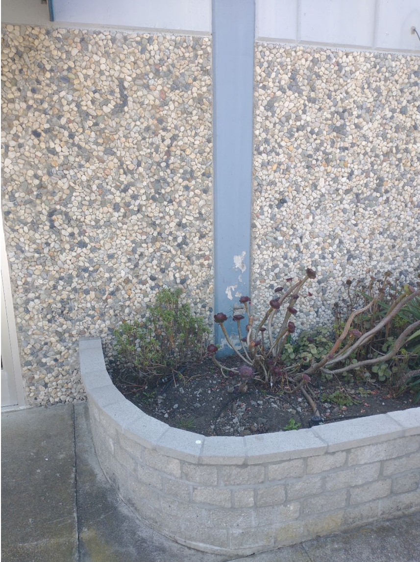
C-3. Planter box and north elevation wall on Brighton Road, detail of the variegated, smooth aggregate set into tilt-up concrete bays and a concrete post, view to the south. Photograph by Yarbrough Architectural Resources, Sept. 15, 2021.
