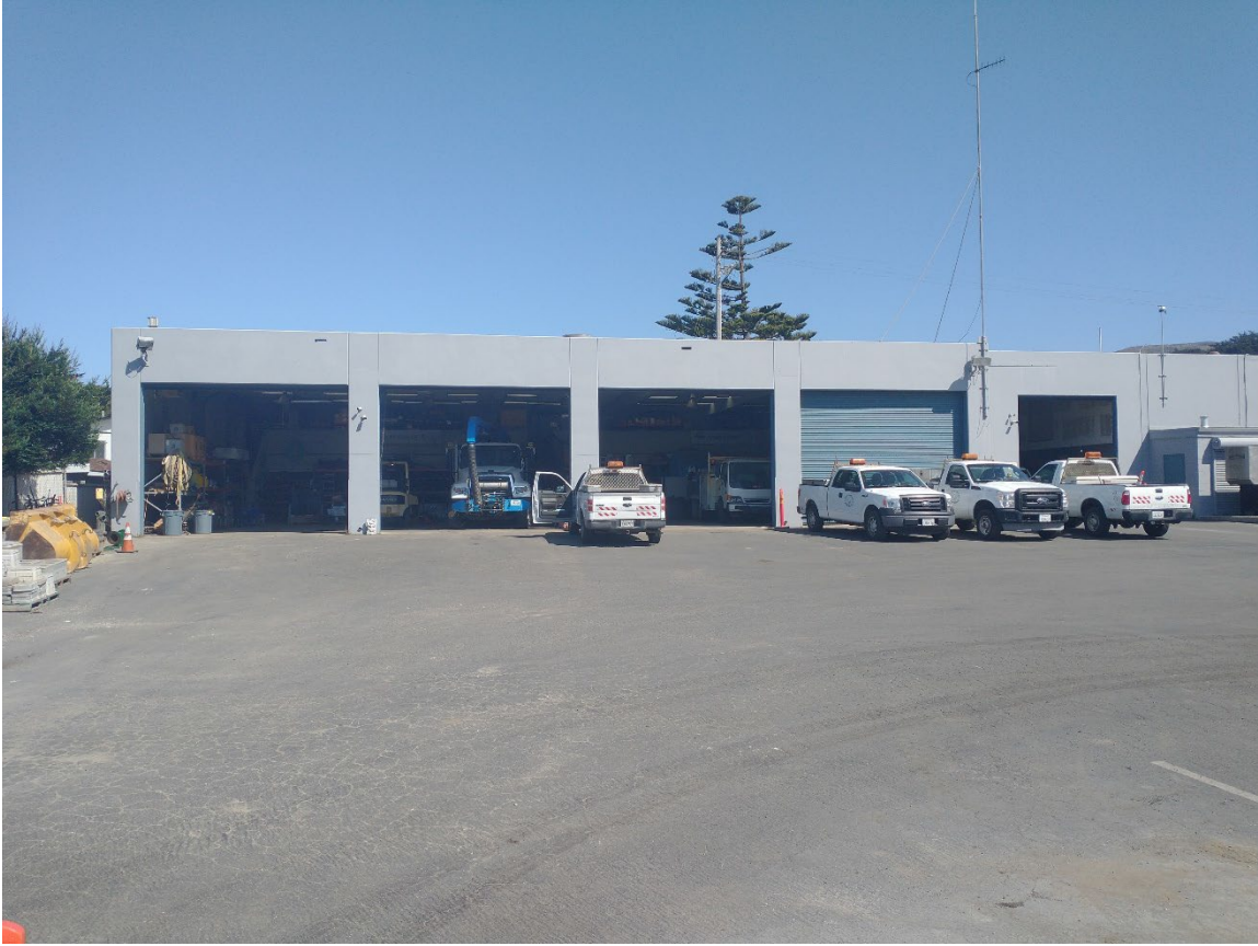
C-9. Left four oversized bays of Building No. 2/Maintenance No. 2 with one garage bay at right for Maintenance No. 1, south elevation, viewed to the north. Photograph by Yarbrough Architectural Resources, Sept. 15, 2021.
