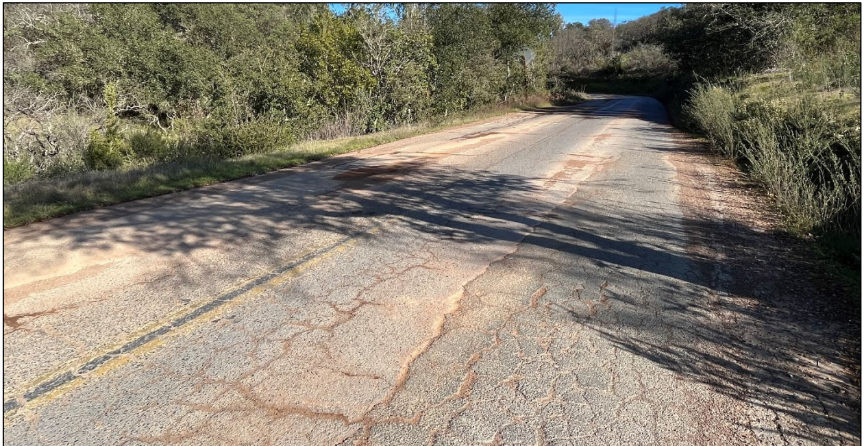
Wood Valley Road (Road ID: 55042) - End of County Maintained Road to Lovall Valley Road, Sonoma. Length: 1.08 Miles. Treatment: Asphalt Overlay
