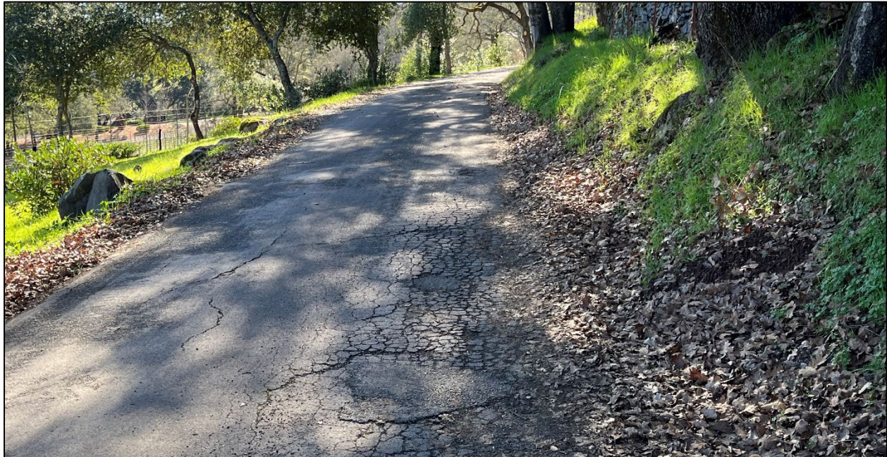
Schultz Road (Road ID: 66064) - Bristol Road to Lawndale Road, Kenwood. Length: 1.24 Miles. Treatment: Asphalt Overlay
