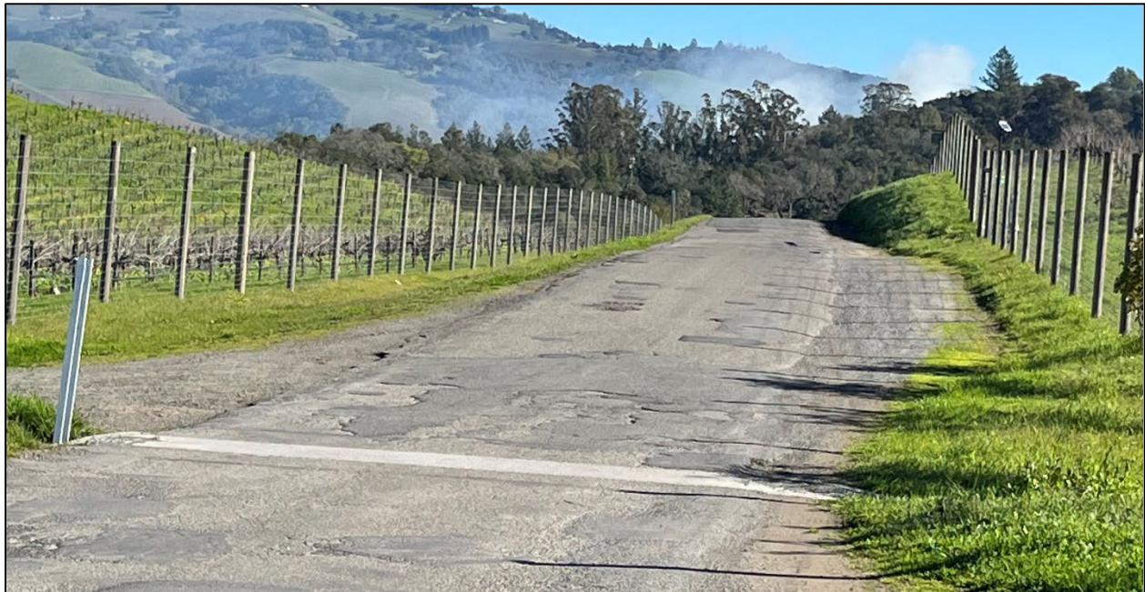
Lawndale Road (Road ID: 76023) - Warm Springs Road to Schultz Road, Kenwood. Length: 1.72 Miles. Treatment: Asphalt Overlay
