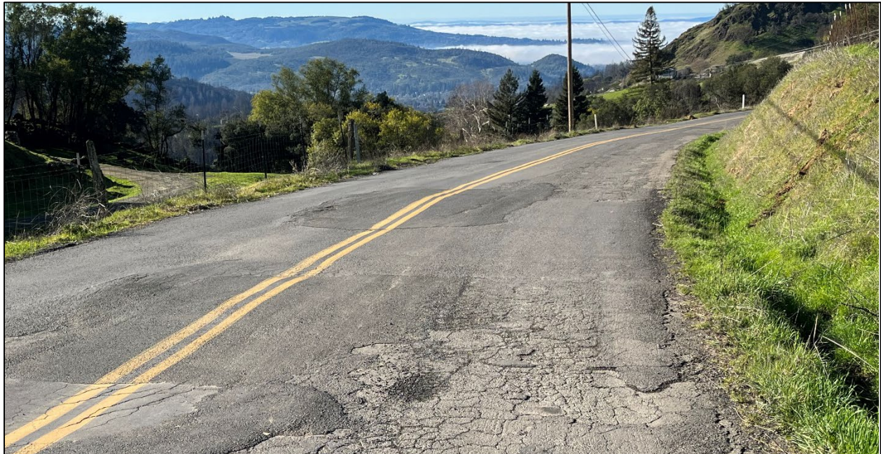
Los Alamos Road (Road ID: 77005) - City of Santa Rosa Limits to End of County Maintained Road, Santa Rosa. Length: 4.06 Miles. Treatment: Asphalt Overlay
