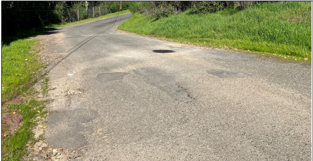
Moon Mountain Drive (Road ID: 66031) - Highway 12 to End of County Maintained Road, Sonoma. Length: 1.52 Miles. Treatment: Asphalt Overlay
