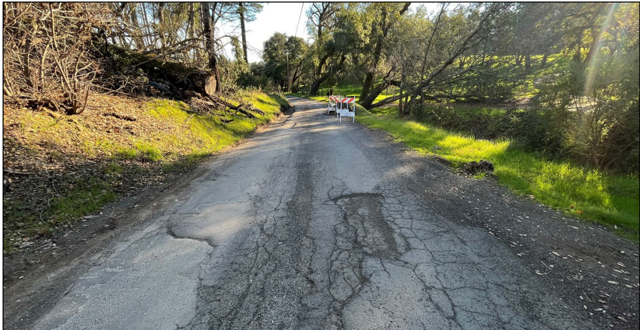
Nelligan Road (Road ID: 66059) – Nuns Canyon Road to End of County Maintained Road, Glen Ellen. Length: 2.20 Miles. Treatment: Asphalt Overlay
