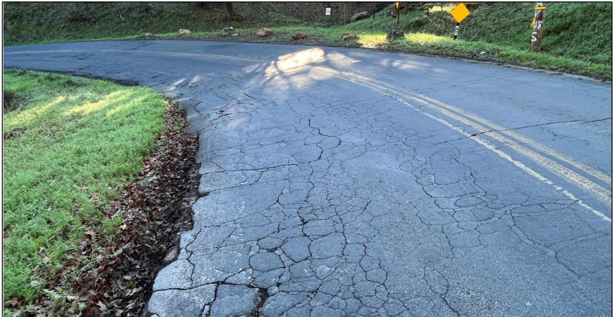
Riebli Road (Road ID: 88001) - Hidden Hills Drive to Wallace Road, Santa Rosa. Length: 0.91 Mile. Treatment: Asphalt Overlay
