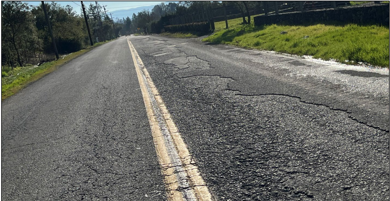
Lovall Valley Road (Road ID: 55040B) - Seventh Street E to Napa County Line, Sonoma. Length: 2.95 Miles. Treatment: Asphalt Overlay
