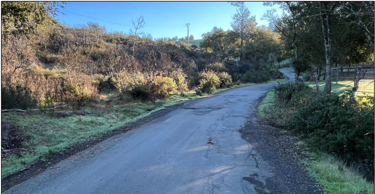
Mountain Home Ranch Roach (Road ID: 87002) - End of County Maintained to Petrified Forest Road, Calistoga. Length: 2.05 Miles. Treatment: Asphalt Overlay
