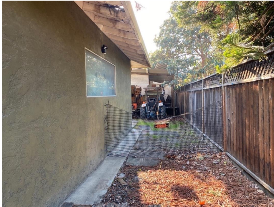
Figure 8. Northwest elevation of 905 N. Capitol Avenue.
