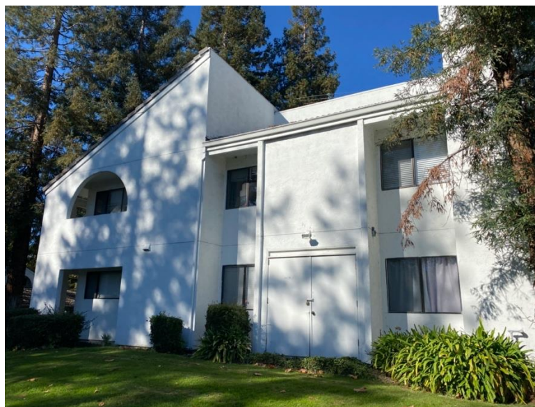
Figure 19. Building Two, north facade on Courtyard Berryessa.
