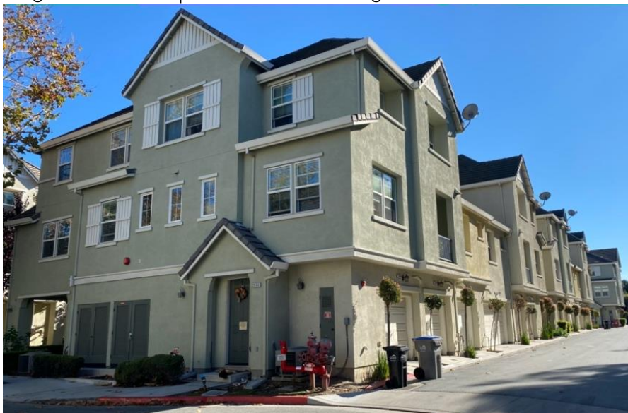
Figure 21. West Corner of Heron Court and Heron Court.
