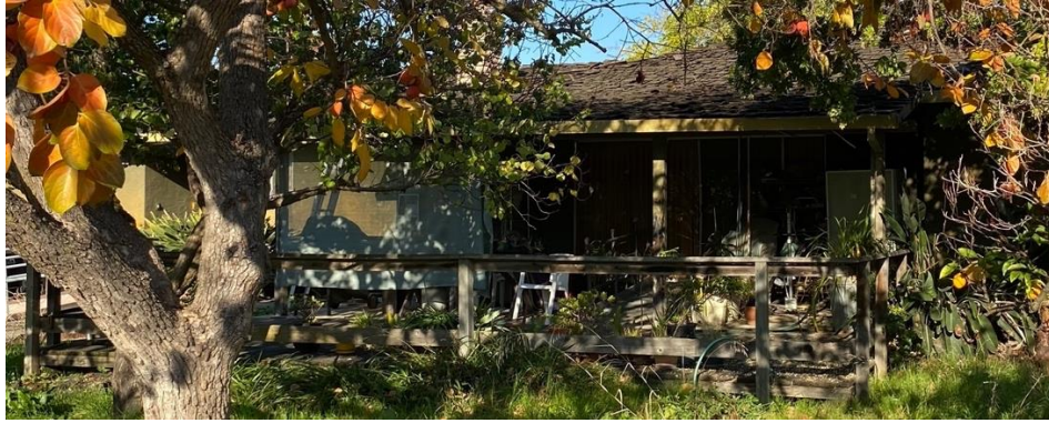
Figure 5. Porch on the rear (southwest) façade of 905 N. Capitol Avenue.
