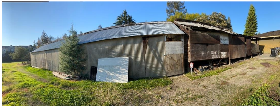
Figure 9. East façade of the shed.
