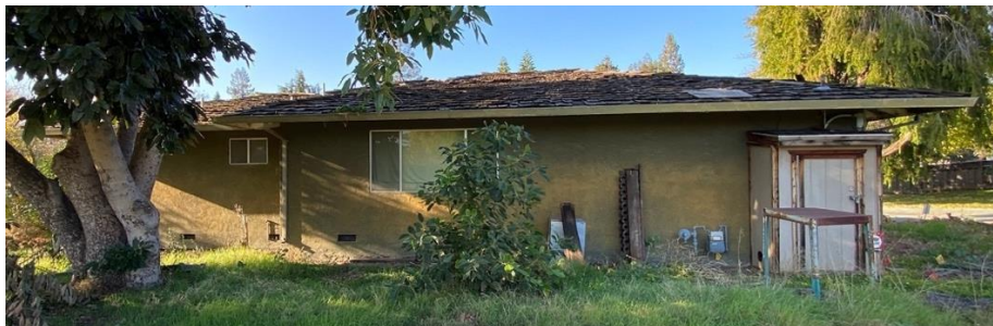
Figure 4. Side (southeast) façade of 905 N. Capitol Avenue.
