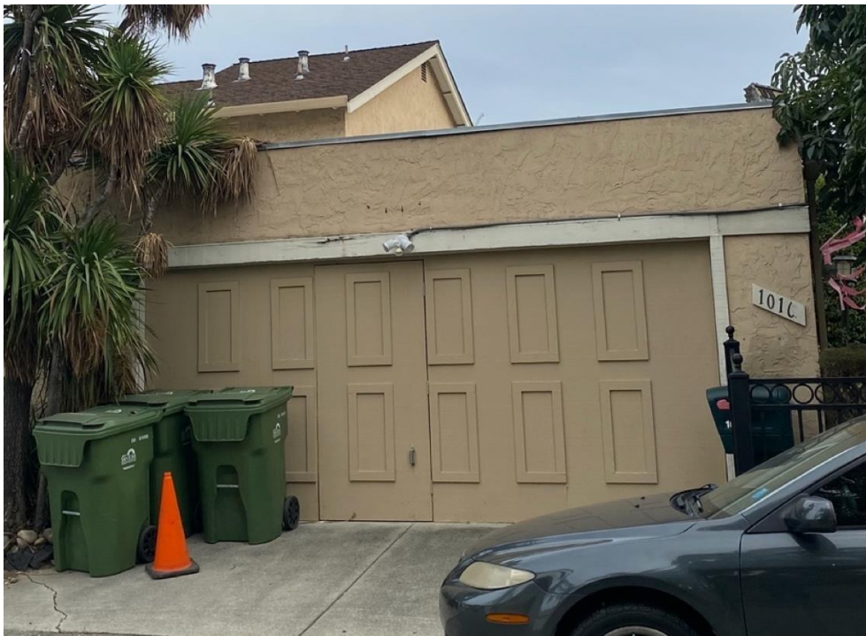
Figure 28. 1016 N. Capitol Avenue. Northwest façade.
