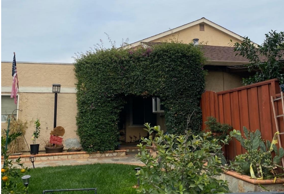
Figure 27. 1016 N. Capitol Avenue. Southwest façade.
