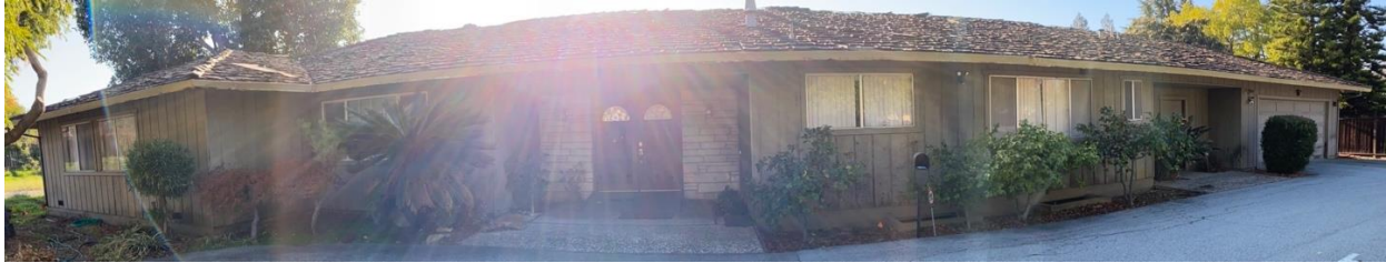
Figure 2. Front (northeast) façade of 905 N. Capitol Avenue.
