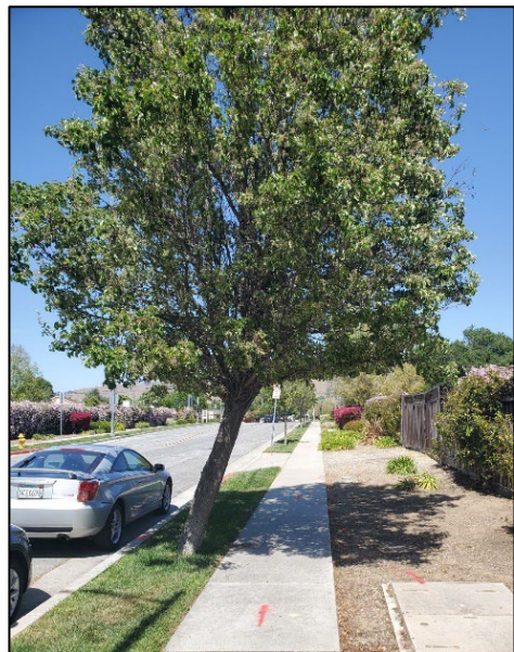
Photo 3 (right): Callery pear #139 had a lean over the sidewalk.
