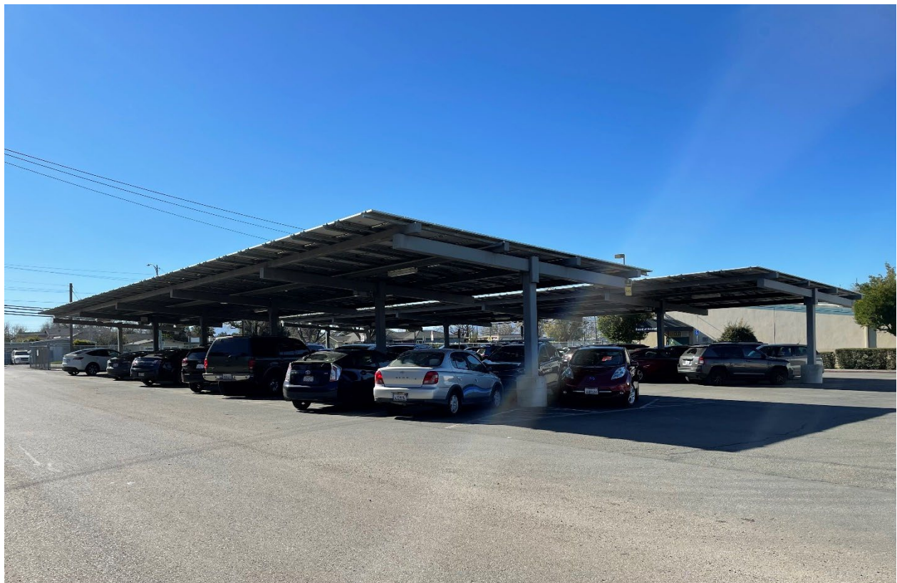
10. Looking southwest at eastern parking lot. Western side to be removed, overall parking lot to remain.
