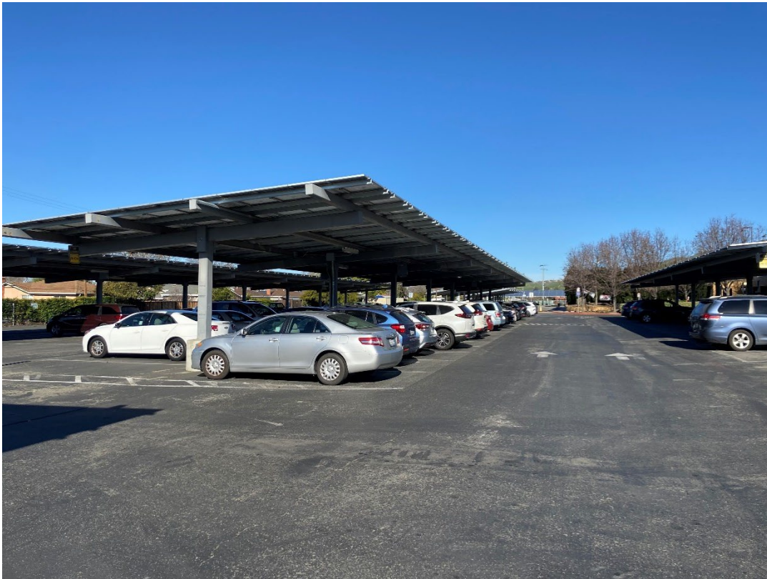
9. Looking north at western parking lot. Central portion to be removed, overall parking lot to remain.
