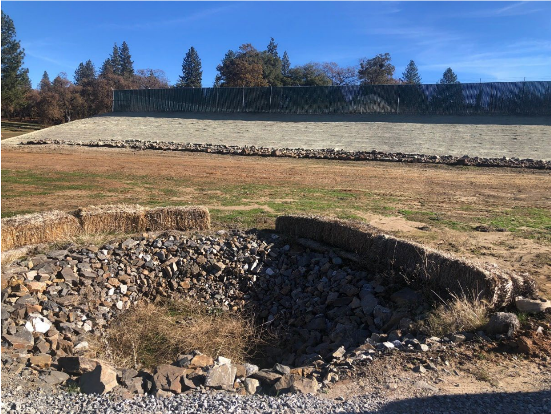
Figure 6: View of spring on APN 16-027-044 with erosion/sediment controls
