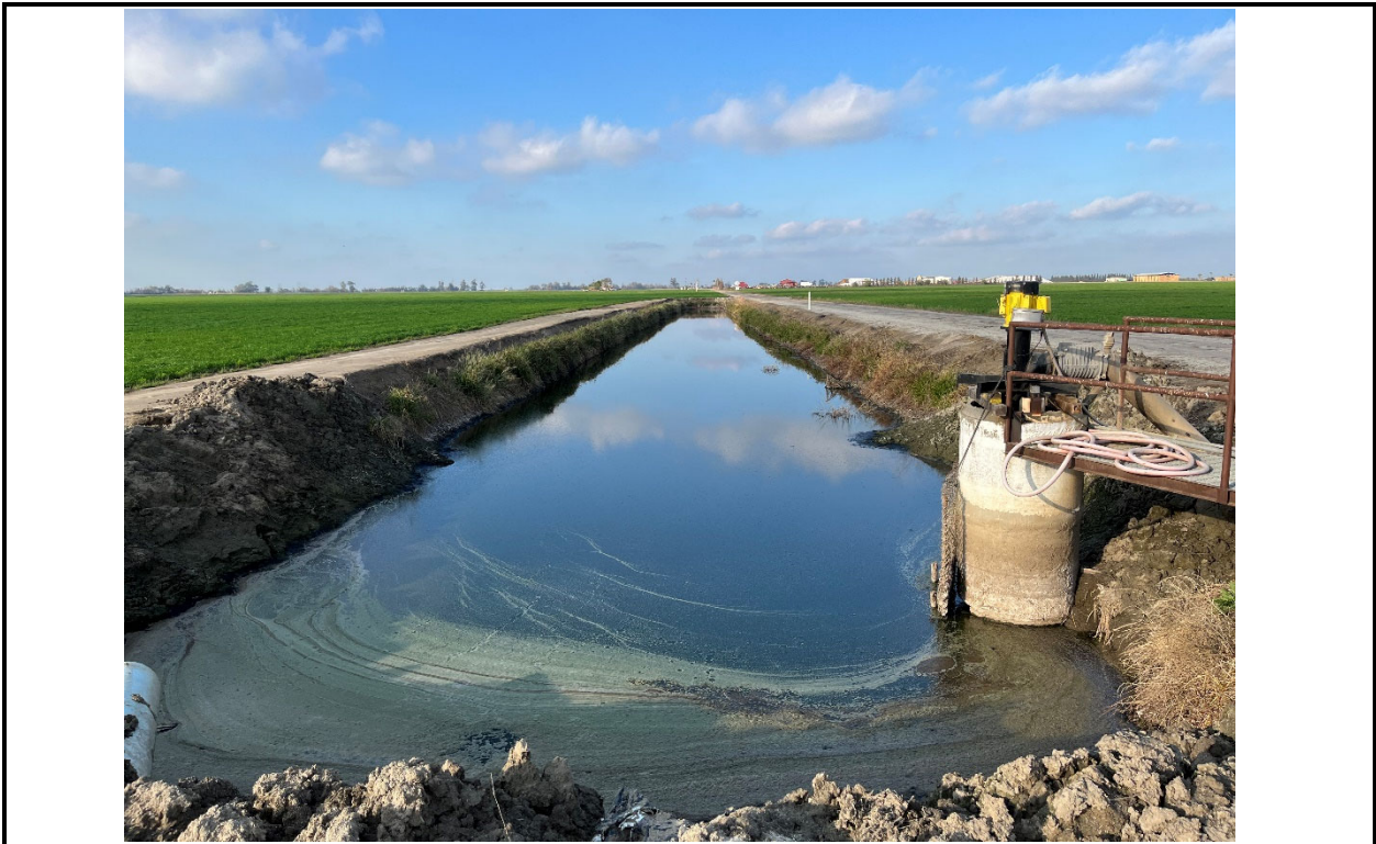
Photo 24. North view of agricultural ditch crossing at alternative pipeline alignment through agricultural field north of Avenue 26 (drainage crossing AD-13).
