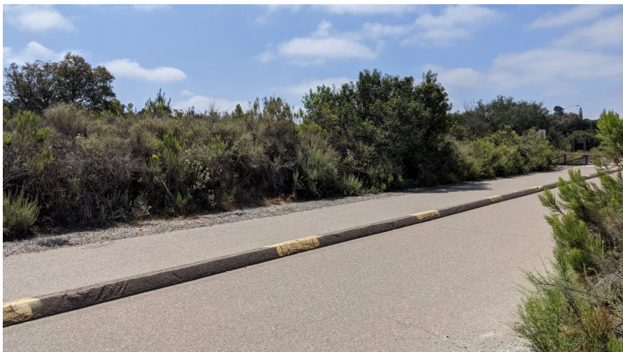
Plate 9. Overview of hill cut at the southern portion of Father Junipero Serra Trail, view to the southeast.
