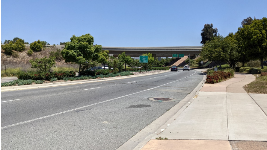
Plate 1. Overview of the APE along Mission Gorge Road, near the SR 52 Overpass, view to the northeast.
