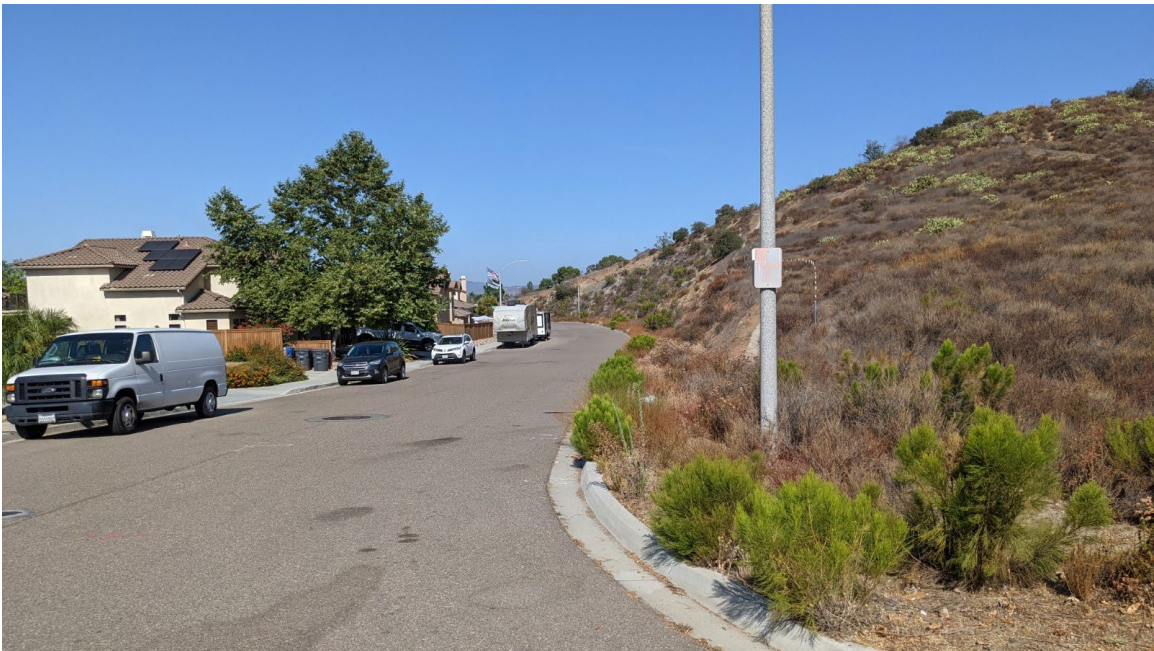
Plate 5. Section of the alignment along Laurel Canyon Road. View to the west.
